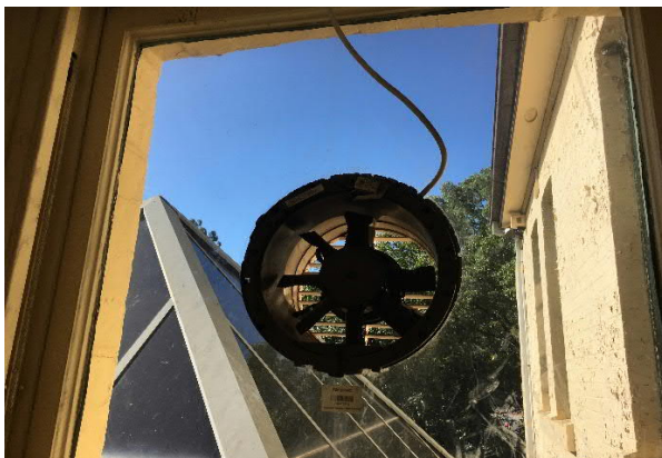
Photo 3. Exhaust fan at Willow Grove is completely sealed in window.
