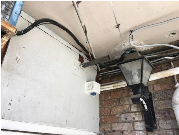
Photo 15. The exterior of 42 Phillip Street was inspected in areas with pipes entering the building to check holes and crevices as possible points of entry. No entry points were detected at this building.
