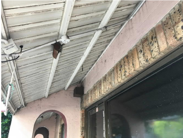
Photo 11. The external structure was intact and sealed offering no entry points for microbats at St George's Terrace.
