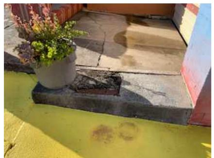
Plate 9 – Another potential set of dip and fill points associated with a UST in front of the metal shed on Lot 2.
