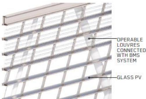
9.8 FIGURE 5 - WT-01A EXTERIOR OPERABLE FACADE AT NORTH, WEST SIDES
