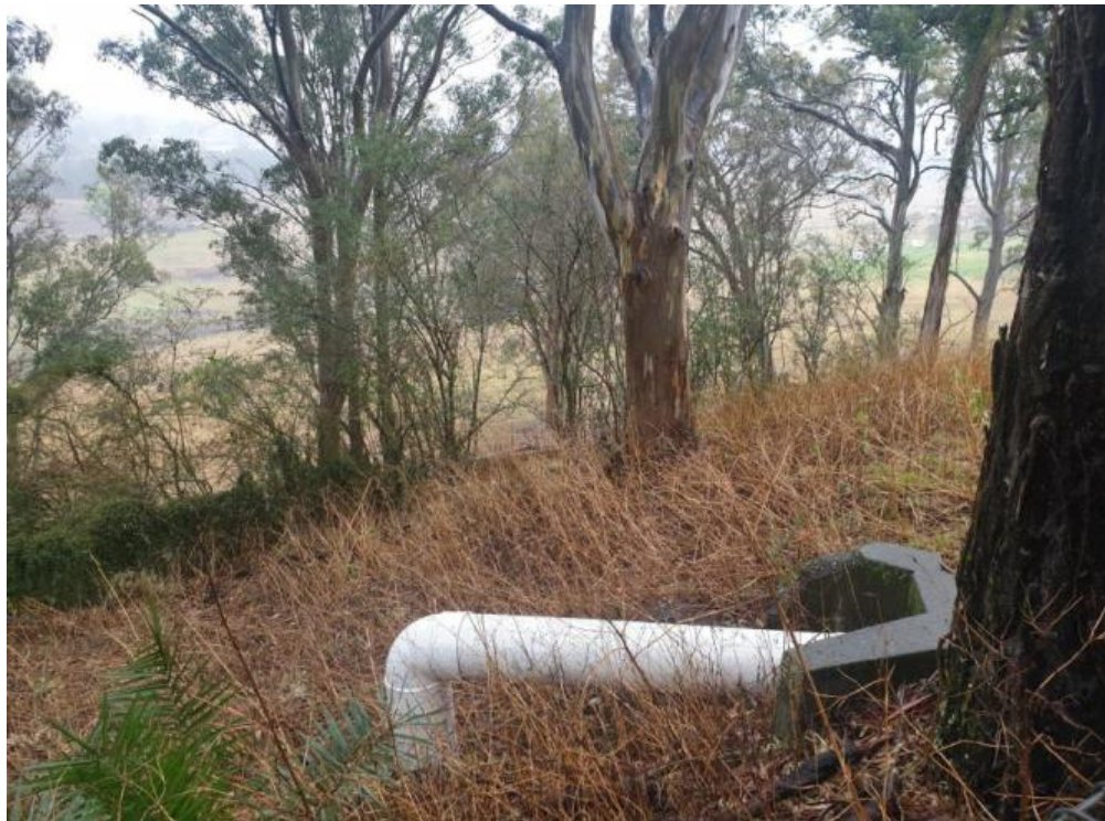
Image 2-8 Existing Headwall and uPVC Diversion Pipe (Bonacci Site Visit on 17.09.2019)
