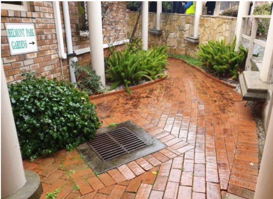
Image 2-6 Existing Stormwater Surface Inlet Pit (Bonacci Site Visit on 17.09.2019)
