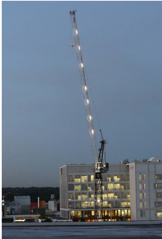
Figure 15: Luffing crane illumination
