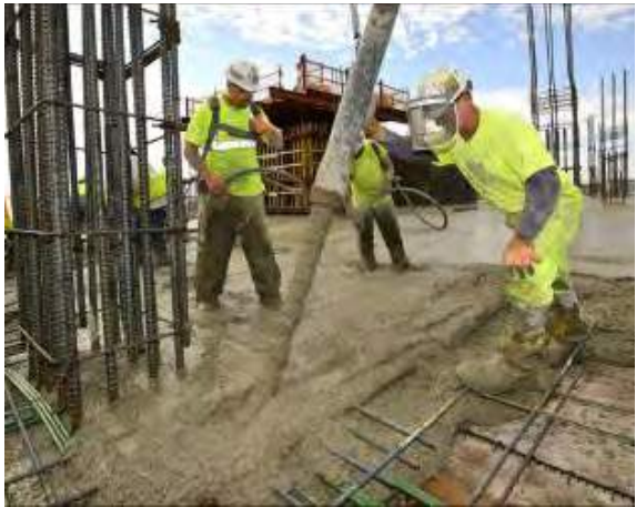
Concrete that has reduced portland cement content, a percentage of captured or reclaimed water and alternate aggregate materials
