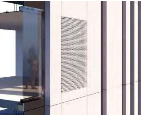
Facade system that minimises heat load and heat loss through the use of shading devices, performance glazing and high performance insulated wall panels
