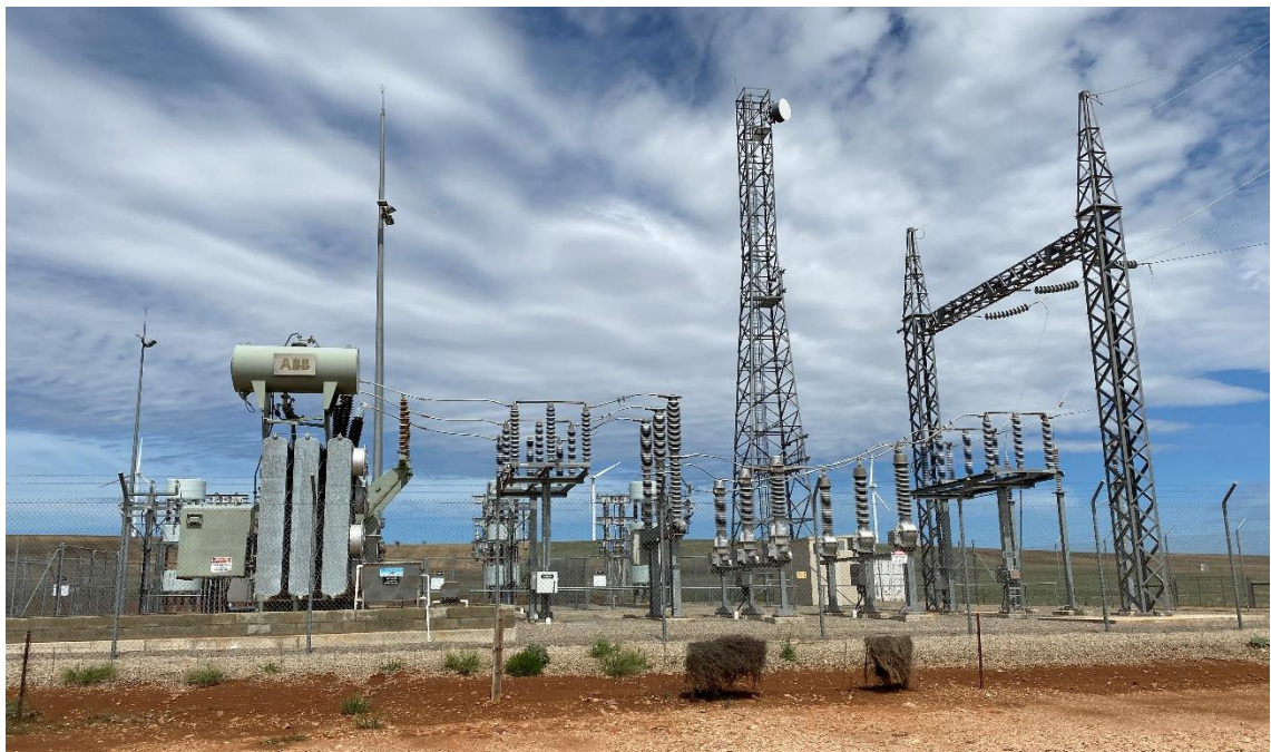
Image 3-7 132 kV switchyard at Clements Gap Wind Farm
