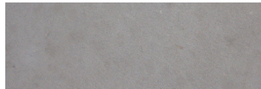
③ Off-form Concrete
