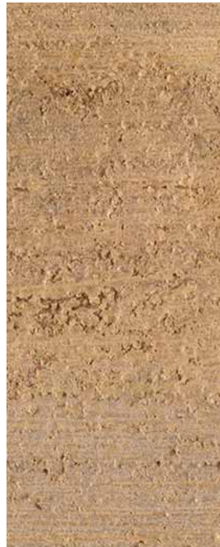
③ Concrete Wall Finish Type 3
