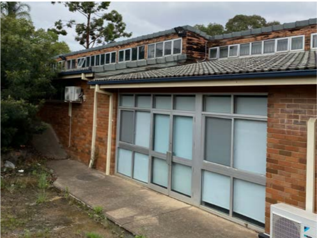
Substantial weathering to eastern highlights and cladding
