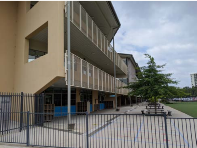
Perforated mesh screen + balustrades
