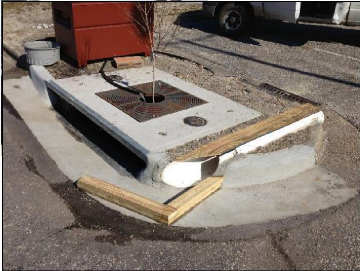
Figure 1. A typical Filterra site with overflow bypass pipe (Anderson and Smolek, 2015).
