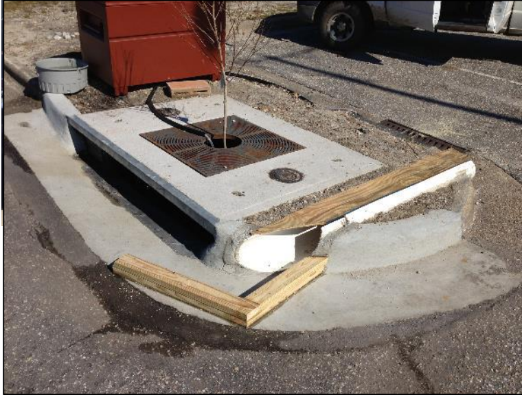
Figure 20. Filterra Site with overflow bypass pipe
