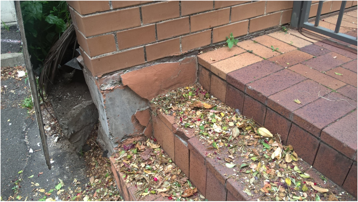
Photo taken at William Lane, at the three steps of the courtyard, showing damaged retaining wall behind the timber board.
