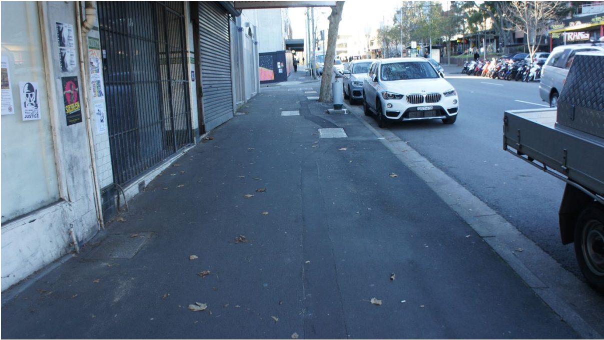
Regent Street Footpath– (looking north)
