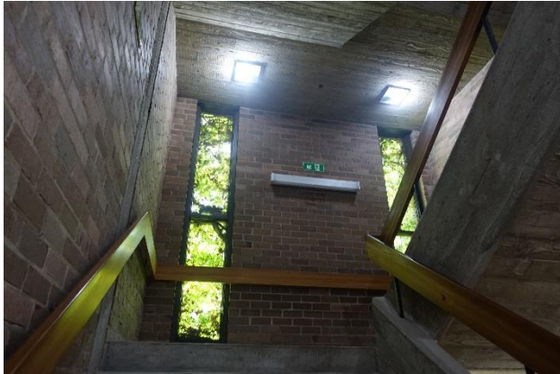
Photo 1 – Load bearing brickwork walls
