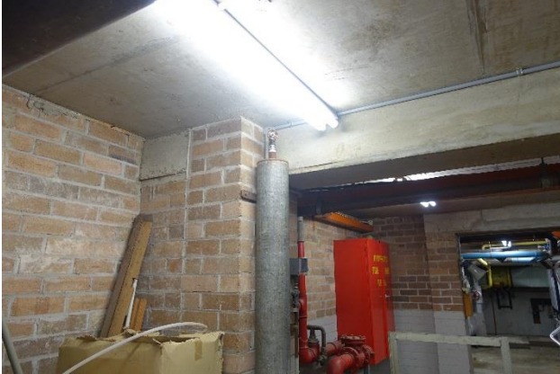
Photo 1 – Load bearing brickwork walls and piers
