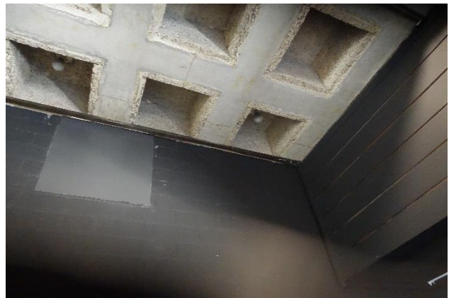
Photo 2 – RC waffle slab on brickwork wall bearing
