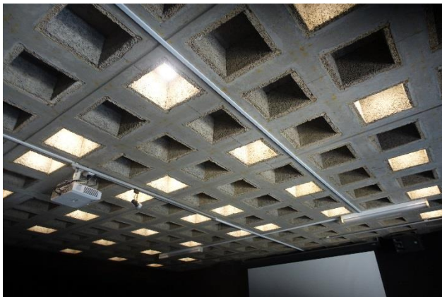
Photo 1 – Level 1 RC waffle slab
