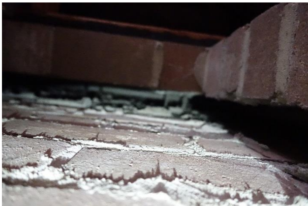
Photo 3 – Brickwork ties in cavity wall [1]
