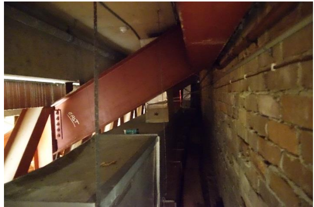
Photo 4 – BT1 truss to raker beam connection
