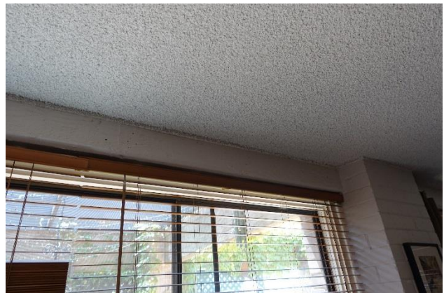
Photo 6 – Typical load bearing brickwork pier
