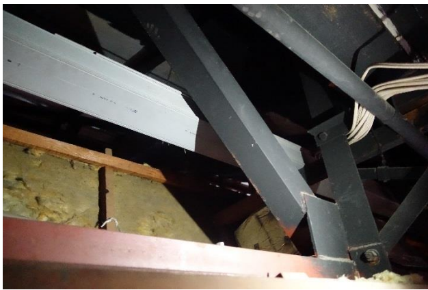
Photo 7 – Roof truss diagonal member
