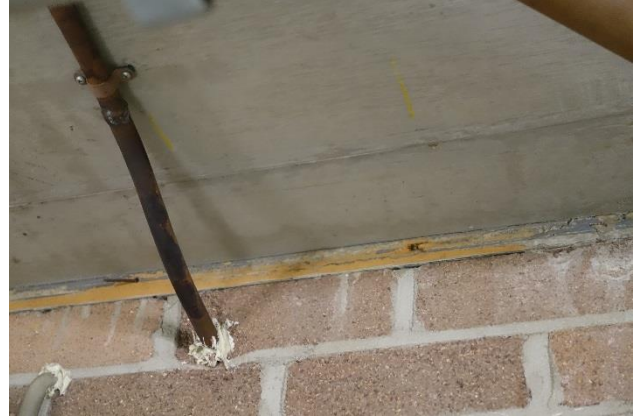
Photo 2 – Typical brickwork damp-proof courses
