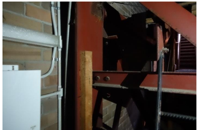
Photo 4 – Roof truss to column bottom connection
