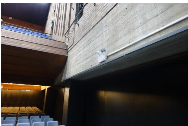
Photo 1 – RC perimeter beam and concrete encased steel columns
