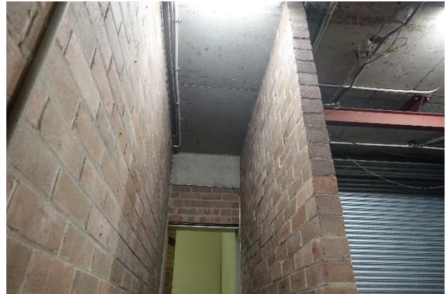
Photo 2 – Typical non-load bearing brickwork wall
