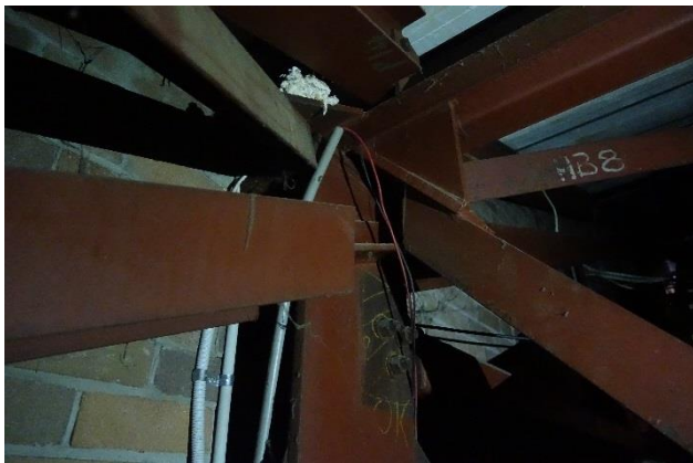
Photo 3 – Roof truss to column top connection
