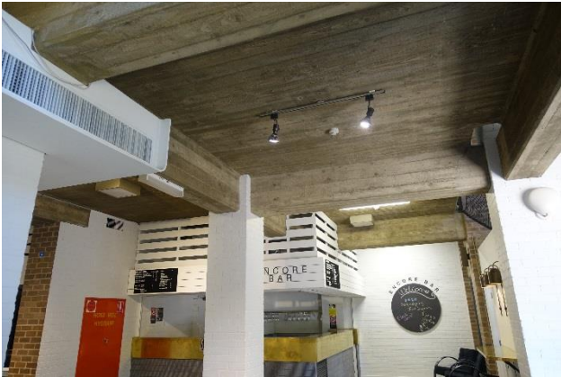
Photo 1 – Foyer RC floor framing [1]
