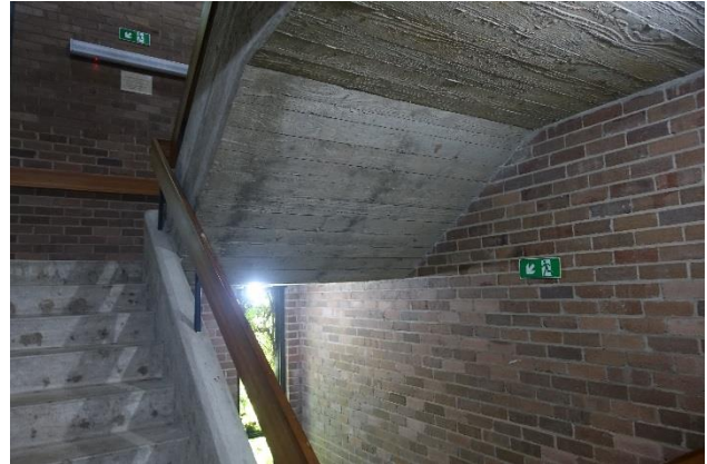
Photo 2 – RC flight and landing slabs
