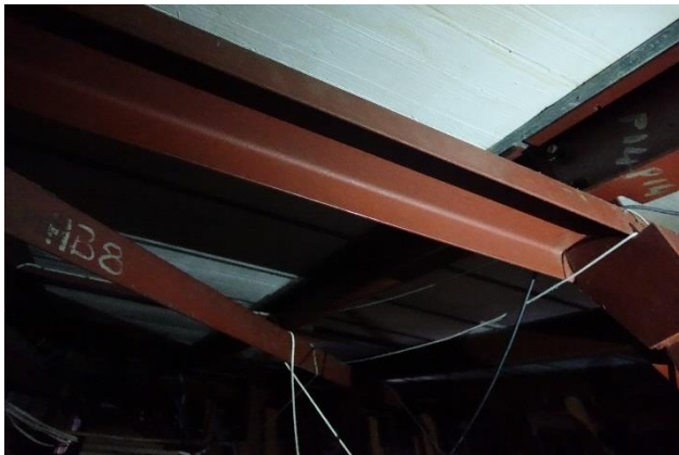
Photo 5 – Roof truss top chord
