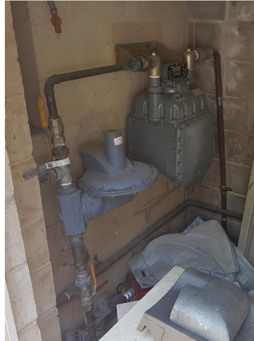
Photo H8 – Existing Volume Gas Meter Assembly
