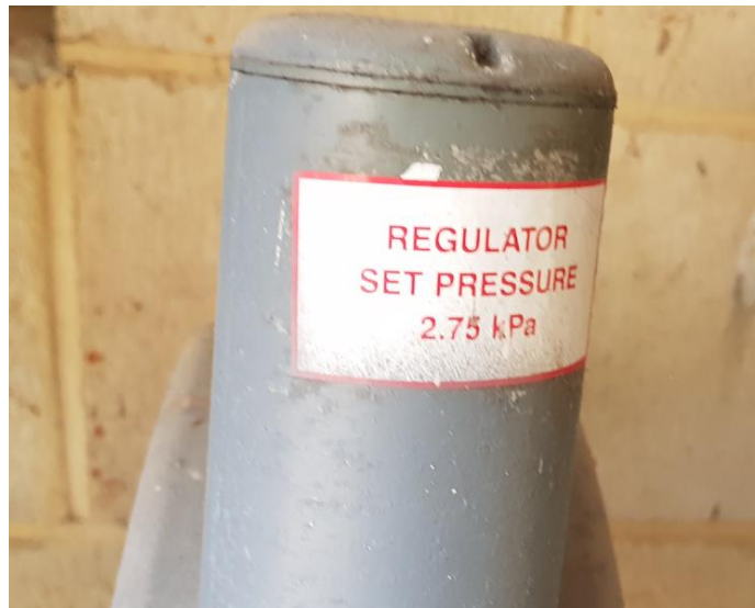
Photo H9 – Existing Gas regulator at meter assembly set to 2.75kpa supply pressure to building
