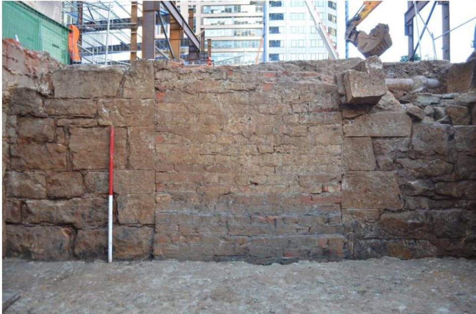
Figure 7: The eastern wall of Cellar 2, showing a bricked-up doorway. Note the substantial stones on either side of the doorway. View to east, scale 1m. DSC_1504
