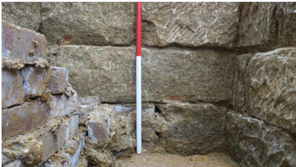
Figure 6: Sandstone blocks in situ within House 42/44 cesspit. IMG_7844. A number of these broke up during demolition.
