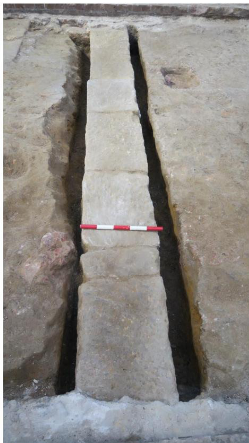
Figure 3: Rear wall footing of House 42. Scale 500mm. IMG_7575.
