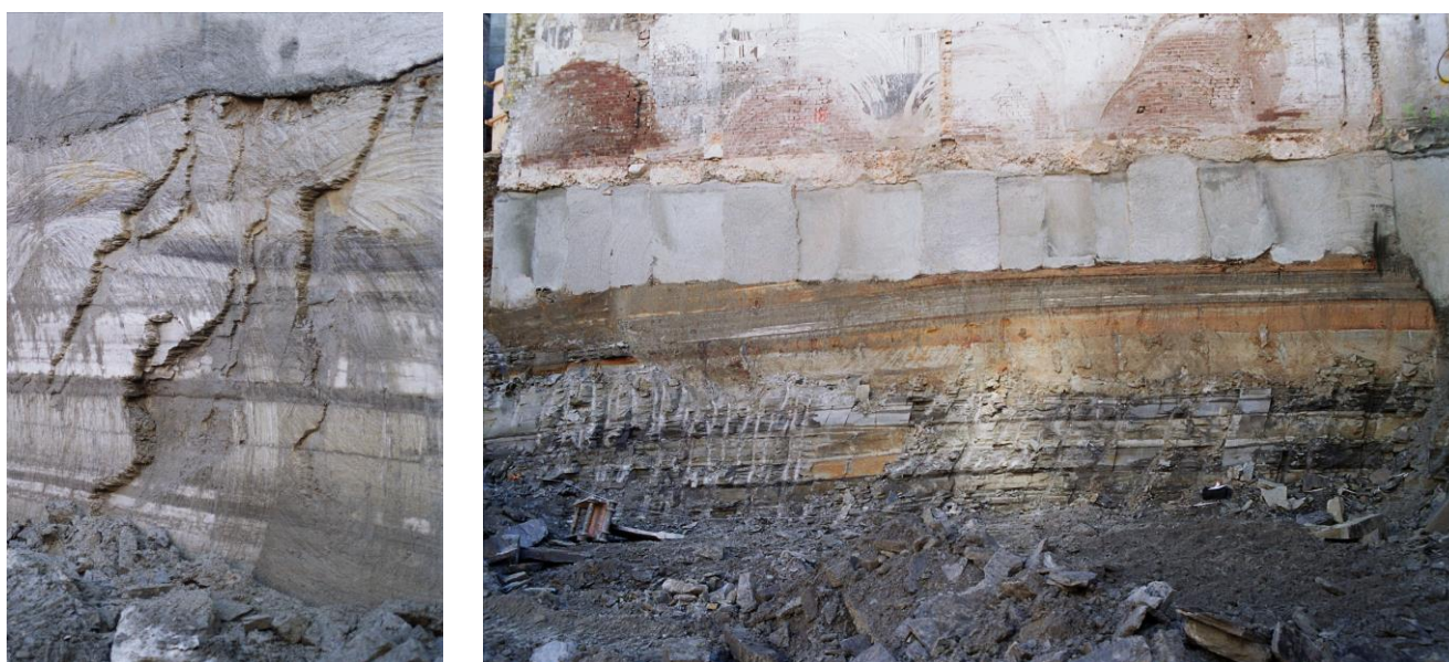
Photo 1: Martin Place Joint Swarm Exposed in A Basement Excavation in The Sydney CBD
