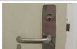
The above image indicates a privacy latch set provided to accessible WC facilities as viewed from the outside
