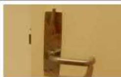
The above image indicates a privacy latch set provided to accessible WC facilities as viewed from within the facility
