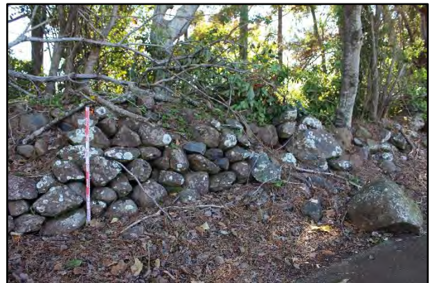
Sample Image 2: Photograph 4 – Detail view of the drystone construction of Wall 1, with scale.
