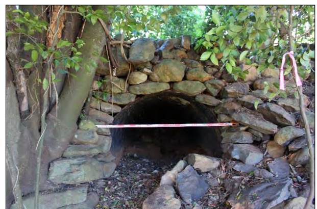
Sample Image 4: Photograph 33 – Detail view of the culvert and surrounding stone work in Wall 3, with scale.
