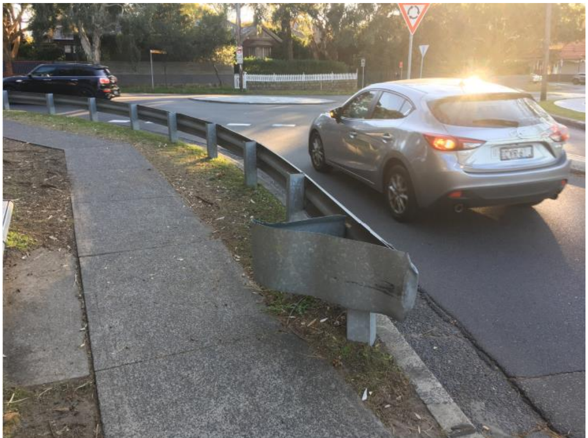
Figure 3-11 Baronga Avenue – Barrier end treatment
