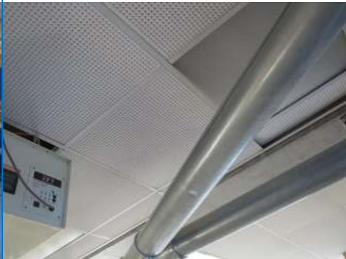
Photo 22: Building C Trades Area Ceiling Tiles. No Asbestos Detected.
