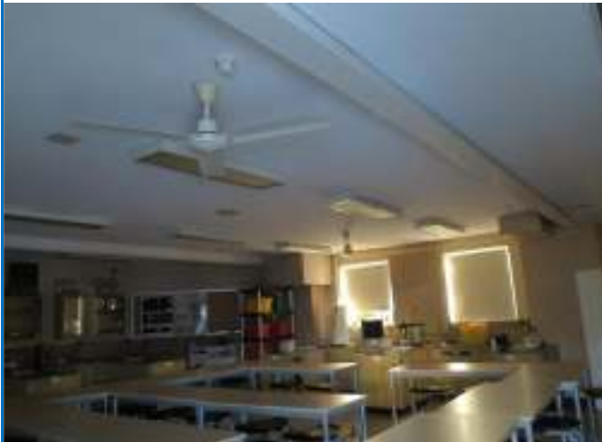
Photo 51: Building J Classroom. Plaster Ceiling. No Asbestos Detected.
