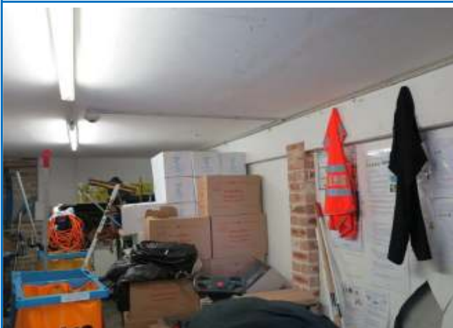
Photo 41: Building E. Lower Level Fibre Cement Wall. No Asbestos Detected.
