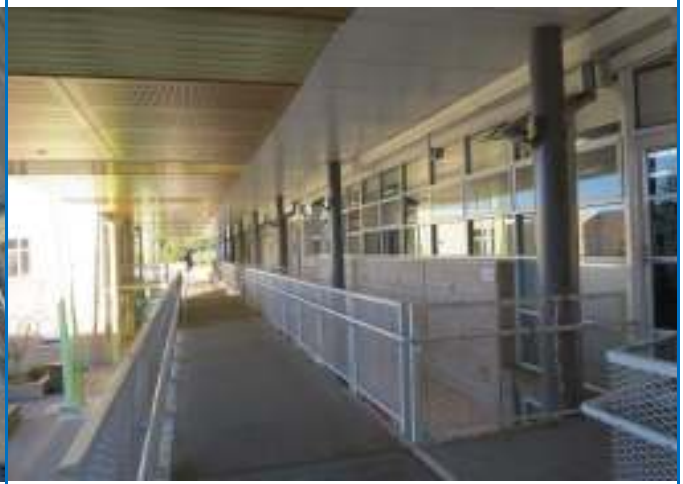
Photo 32: Building D. Upper Level. Awning Fibre Cement & Wood Panel. No Asbestos Detected.
