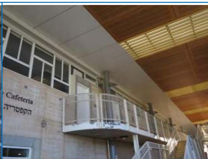
Photo 26: Building D. Fibre Cement & Wood Panel Ceiling. No Asbestos Detected.
