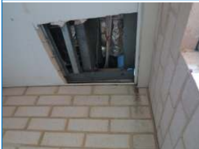
Photo 9: Building A. SMF Detected In The Ceiling Cavity A. No Asbestos Detected.
