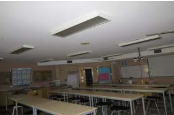
Photo 48: Building J Classroom. Plaster Ceiling. No Asbestos Detected.
