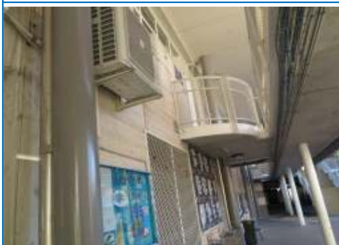
Photo 29: Building D. Concrete Panel Construction. No Asbestos Detected.
