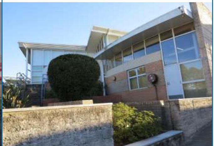
Photo 6: Building A. External Eaves Lined With Fibre Cement. No Asbestos Detected.
