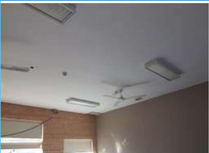
Photo 44: Building E Classroom. Plasterboard Ceiling. No Asbestos Detected.
