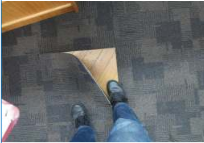
Photo 3: Building A. Wooden Floorboards Under Carpet Squares. No Asbestos Present.
