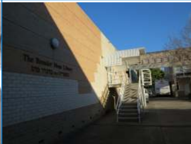
Photo 10: Building A. Awning Over Rear Entry To Library Lined With Fibre Cement. No Asbestos Detected.
