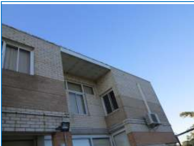
Photo 13: Building B Fibre Cement Awning, Upper Level. No Asbestos Detected.
