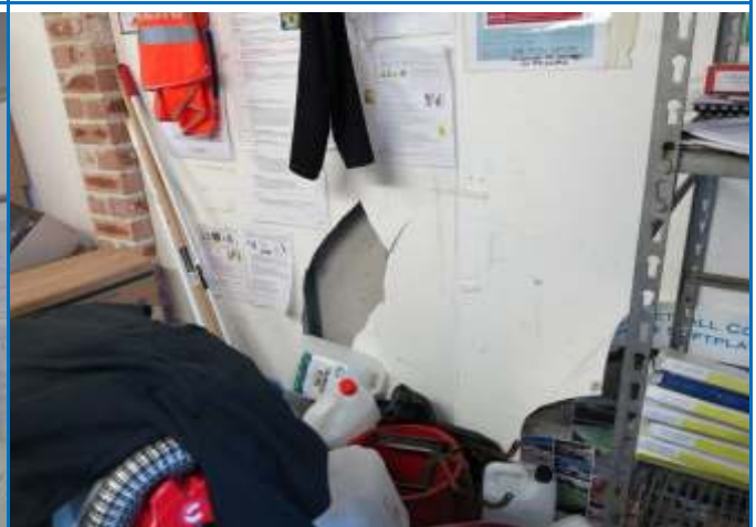
Photo 42: Building E Damaged Fibre Cement Wall Lower Level. No Asbestos Detected.
