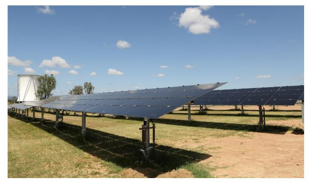
Figure 4-3 Typical single-axis tracking system.
