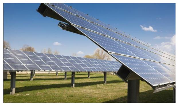
Figure 4-2 Typical fixed tilted system.
