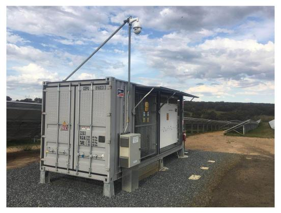
Figure 4-5 Typical illustration of a PCU within the array.
