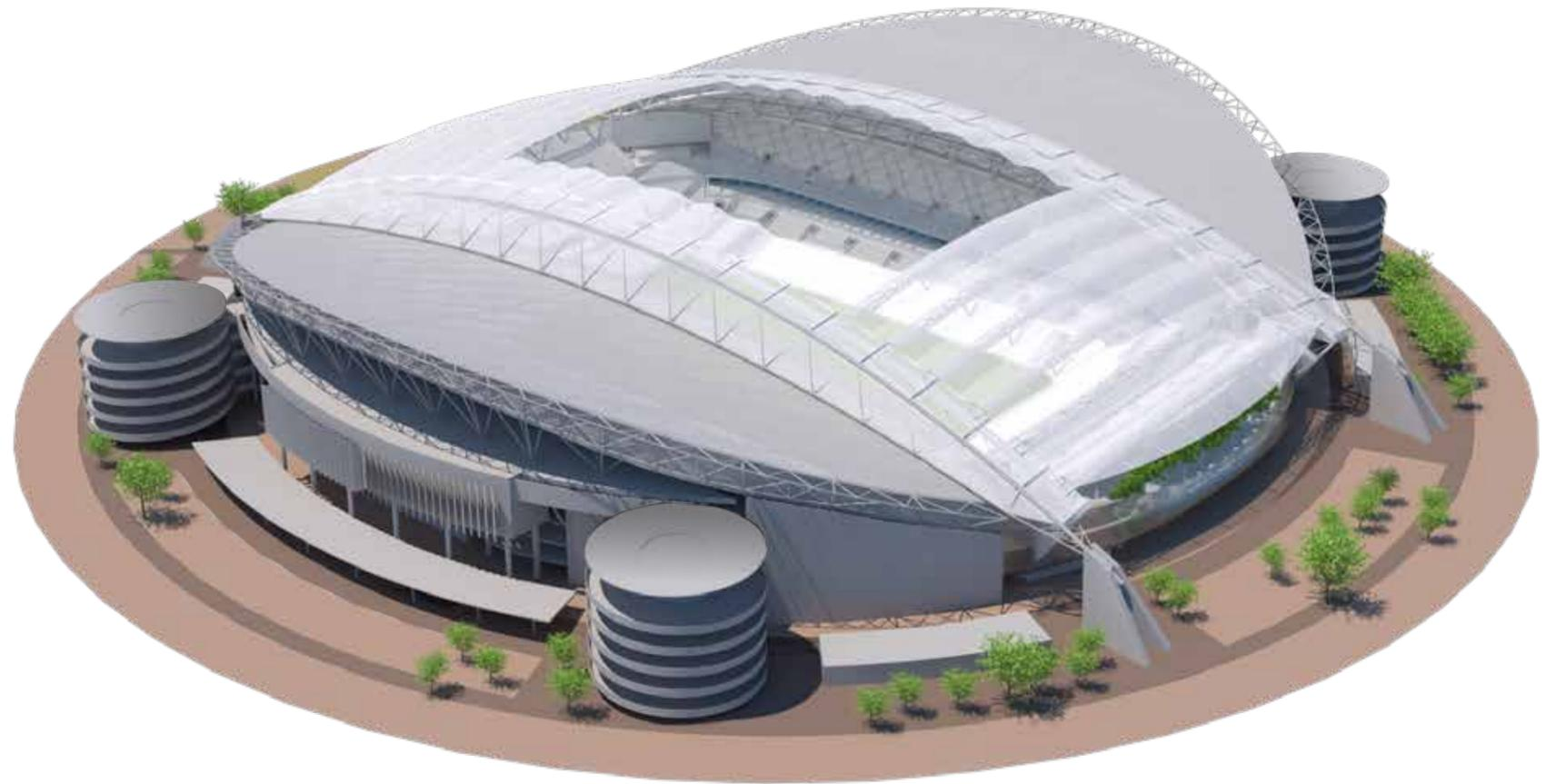
Figure 28: Aerial view of the stadium highlighting the new roof between the existing structural arches.
