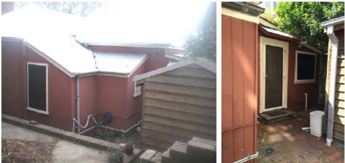
Figure 4.14: Skillion roofed timber weatherboard structures enclosing the bathroom and WC at the rear of the Cottage (left); western wall of the skillion roofed section containing the kitchen and Room 4 at the rear of the Cottage (right). The small shed can be seen in both photographs. (Source: TKD 2016: Fig 71)
