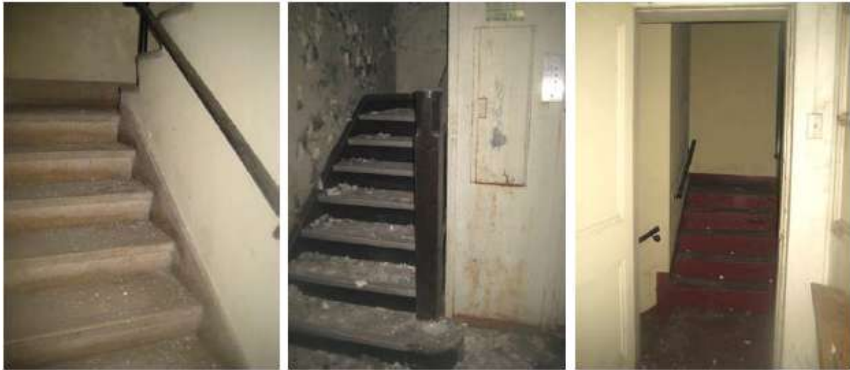
Figure 4.25: Terrazzo stair on the northern side of the building linking the ground and first floors (left), stained and polished timber stair providing access to the residential apartment (centre) and concrete stair connecting all levels of the building, including the roof (right). (Source: TKD 2016: Fig 83)
