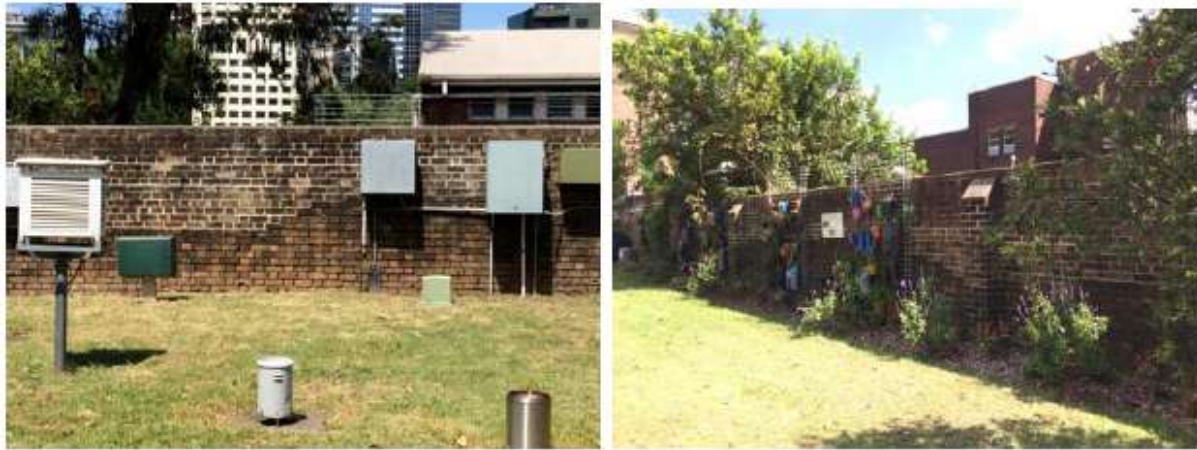
Figure 4.34: Northern section of the wall, to the east of the Messenger's Cottage. Later works associated with the upper sections of the wall are clearly visible (left); southern section of the wall, which is strengthened by brick piers (right). (Source: TKD 2016: Fig 97)
