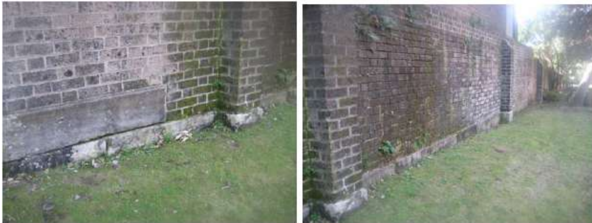
Figure 4.35: The extant brick wall is constructed over stone footings. (Source: TKD 2016: Fig 98)
