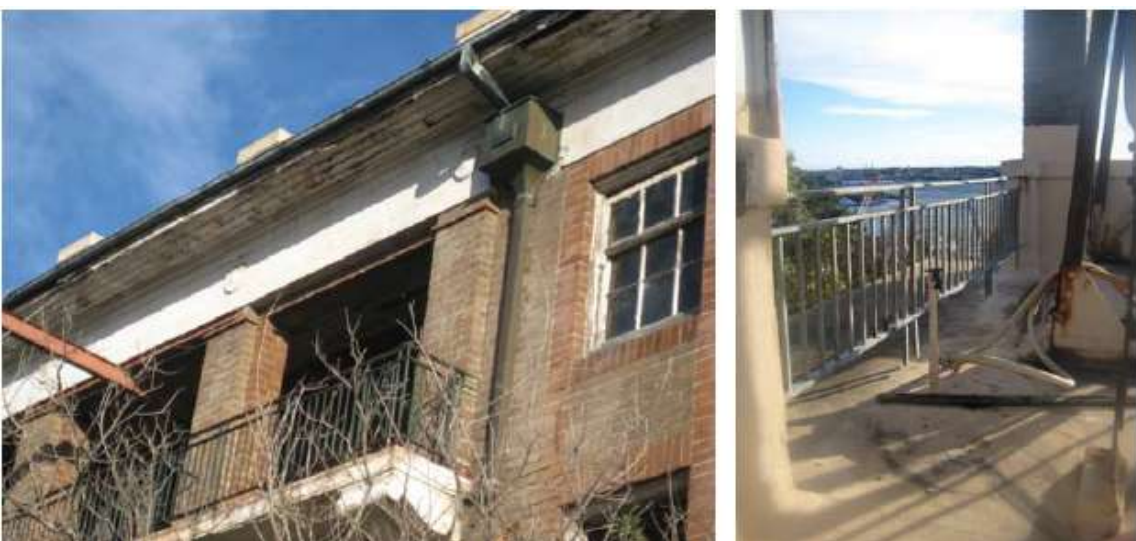
Figure 4.21: Wrought metal balustrade, bracket and piers associated with the second floor loggia. Medallions are located above the piers in the frieze (left). Similar balustrading is located at roof level (right). (Source: TKD 2016: Fig 79)
