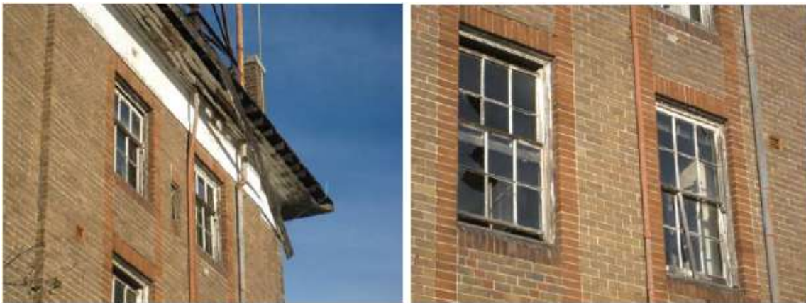
Figure 4.20: Deteriorating eaves fabric (left) and window joinery (right). (Source: TKD 2016: Fig 78)
