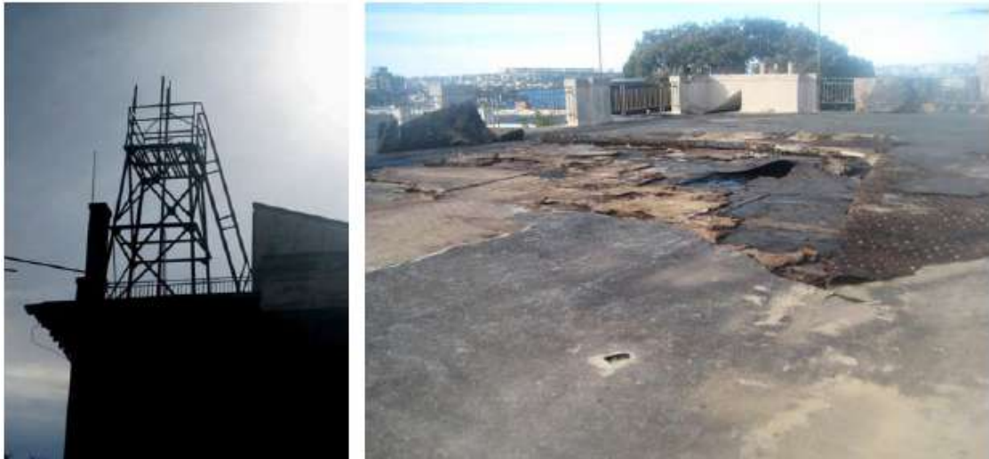
Figure 4.22: Steel-framed tower that was installed to support the wind recording apparatus (left); roof membranes are in very poor condition and are missing in some locations (right). (Source: TKD 2016: Fig 80)
