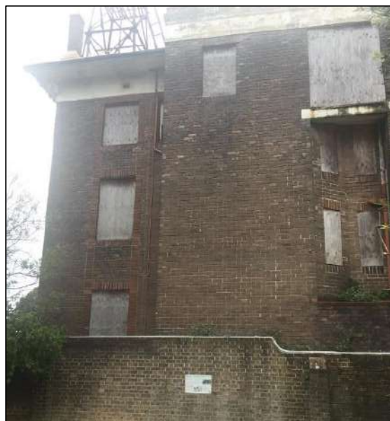
Figure 8.7: Existing southern façade of MET Building. Existing penetrations to be used in new southern bridge connection visible (Source: Curio 2019)
