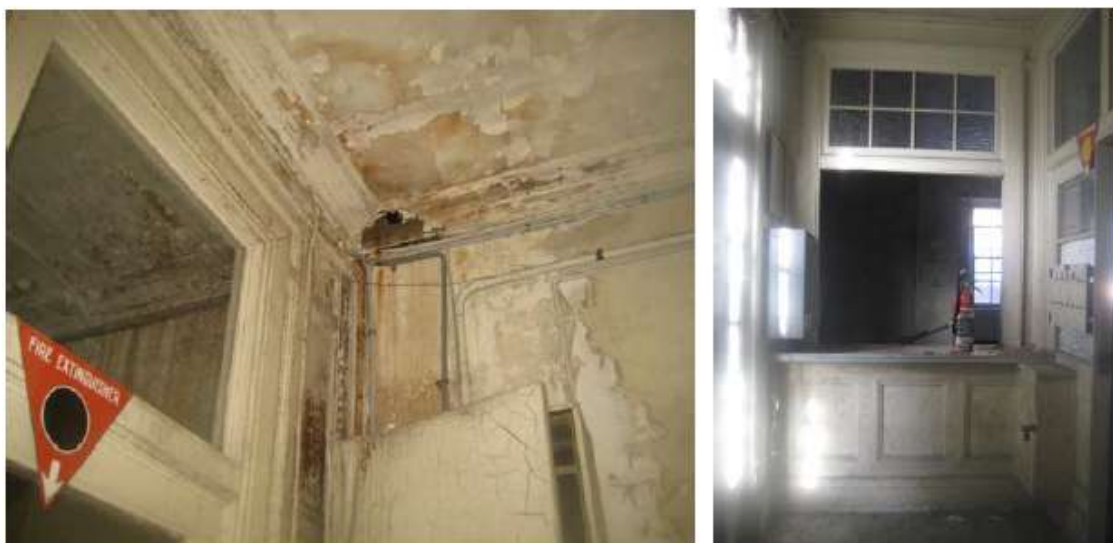
Figure 4.24: Ground floor reception area adjacent to the main entrance. The space has retained a substantial amount of original fabric, including timber joinery items such as the counter and highlight window over it. Decorative plaster cornices are suffering from water damage. (Source: TKD 2016: Fig 82)
