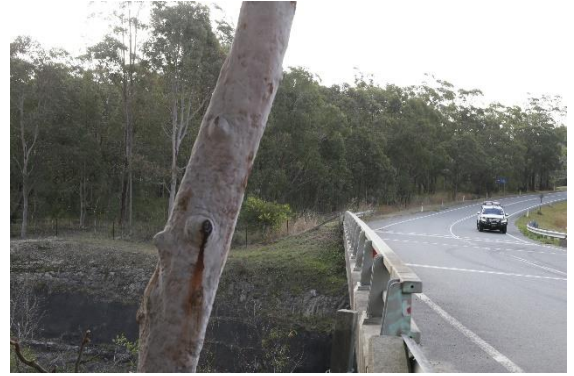
Photograph 4-4 VP6 - Wilton Road at the Bridge over Newstan Eraring Private coal road, looking north-west
