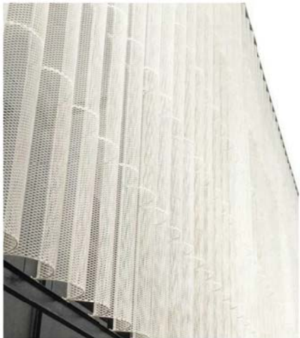
1. PERFORATED SCREEN - ALUMINIUM, FINISH - POWDERCOATED WHITE
