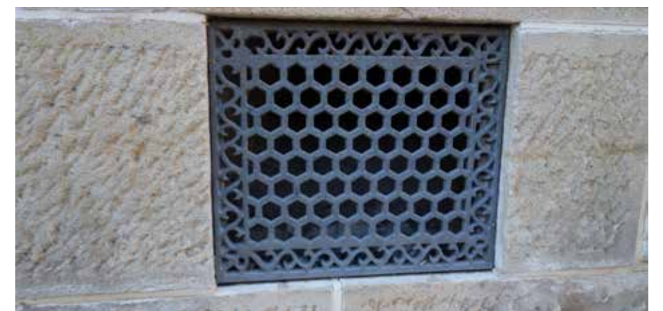
Figure 2.107: Detail of original floor vent located above the plinth course.
