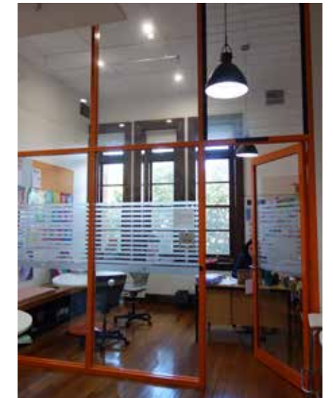
Figure 2.88: Modern partitions to staff offices on Level 3. Note the exposed timber floorboards and battened ceiling.
