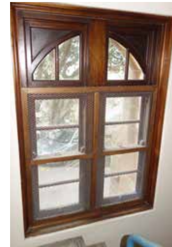
Figure 2.97: Original timber double hung windows with arched highlight over. Note the secondary timber framed meshed screen, resulting in them no longer being operable.
