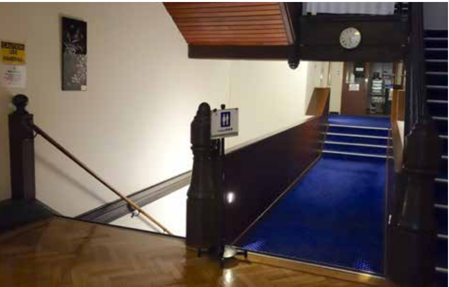
Figure 2.39: Non-original bridge through the main staircase provides access to the Hughes Centre at Level 2.
