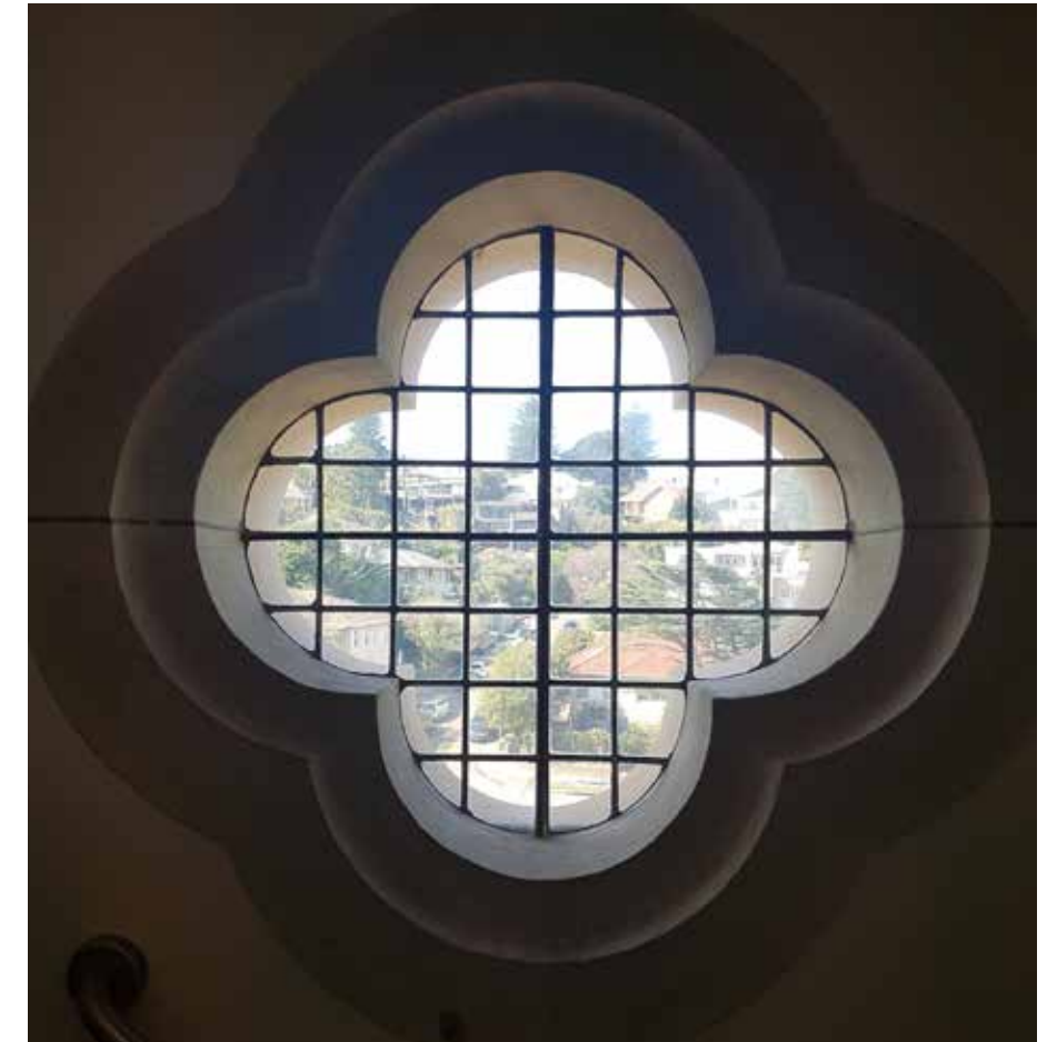
Figure 2.99: Close-up of the quatrefoil shaped window on the eastern elevation of South wing with its stone surrounds and clear, square leaded glass.
