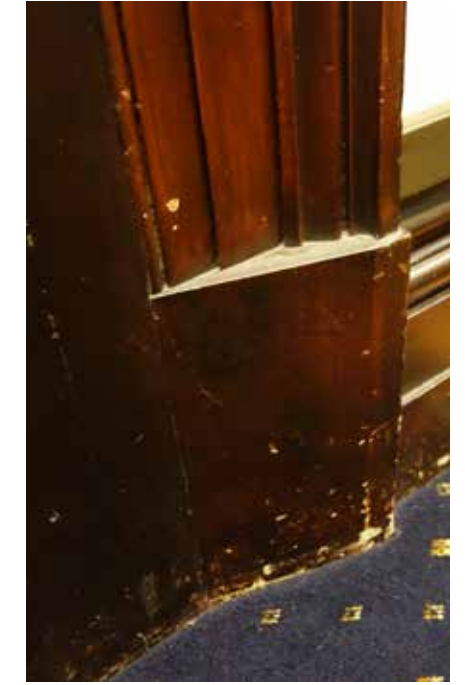
Figure 2.154: Detail of the skirting and architrave profiles on Level 2 at Claremont, likely dating from 1851.
