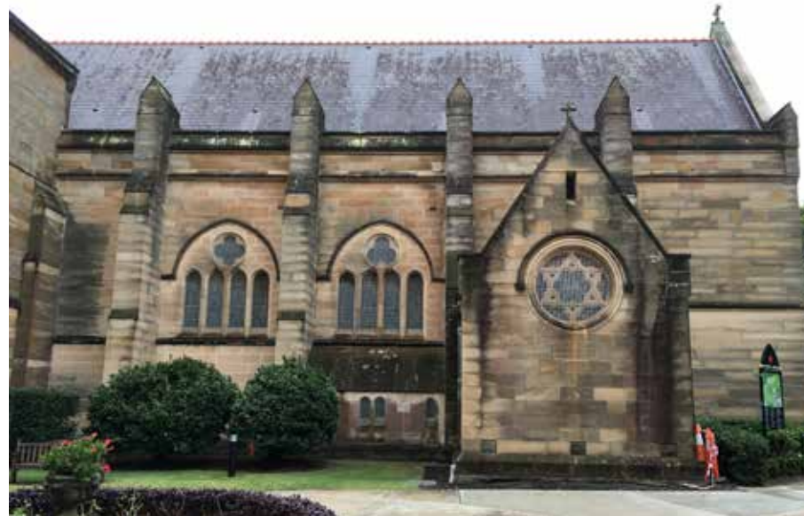
Figure 2.104: Southern elevation of the Chapel, showing the division of the Chapel into bays, defined by the evenly spaced buttresses and the Side / Stranger's Chapel.
