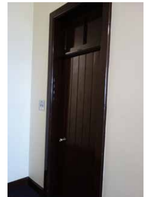
Figure 2.68: Original painted timber boarded doors on Level 5 with highlight over.
