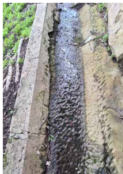
Figure 2.216: Sandstone channel at base of Hunt retaining wall.
