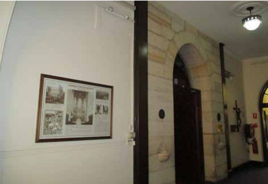
Figure 2.108: The main entry to the Chapel from Level 2 of the Main School building. Note the unfinished sandstone ashlar wall adjacent rendered walls.
