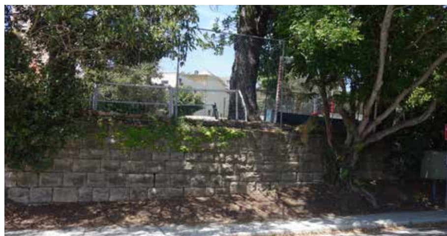
Figure 2.8: Sandstone retaining wall and chain link wire mesh fence at the northern end of the playing fields, close to the corner of Vacluse Road and Gilliver Avenue.
