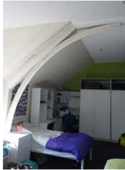
Figure 2.95: Typical bedroom on Level 5 of the South wing. Note the exposed steel roof trusses.
