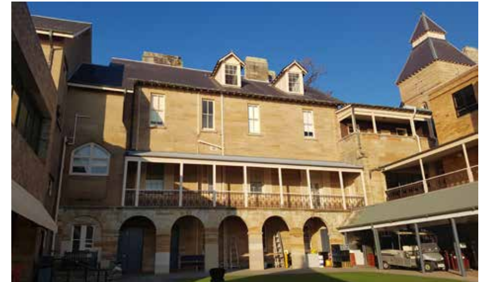
Figure 2.134: Western elevation of Claremont, with the 1851 stone arched loggia (Level 1) and verandah above (Level 2). The Hughes Centre balcony and covered way to Cloister Courtyard are visible to the far right of the image. Level 3 with the four sash windows and the hipped roof were constructed as part of Hunts 1882 remodelling of the building. The dormer windows were added in the 1920s. The timber shingled balcony and rooms behind on Level 3 were added in the 1930s.
