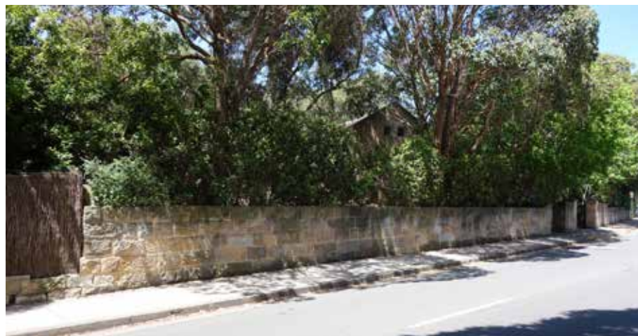
Figure 2.7: Medium height sandstone ashlar wall with picked finish and brushwood fencing surrounding Claremont Cottage on Vacluse Road.
