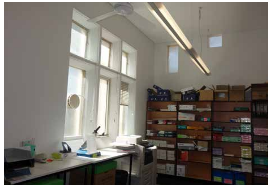
Figure 2.60: A view of the print room on Level 3 with the stepped opaque glass openings on the eastern wall (right), indicating a former stair along this wall.
