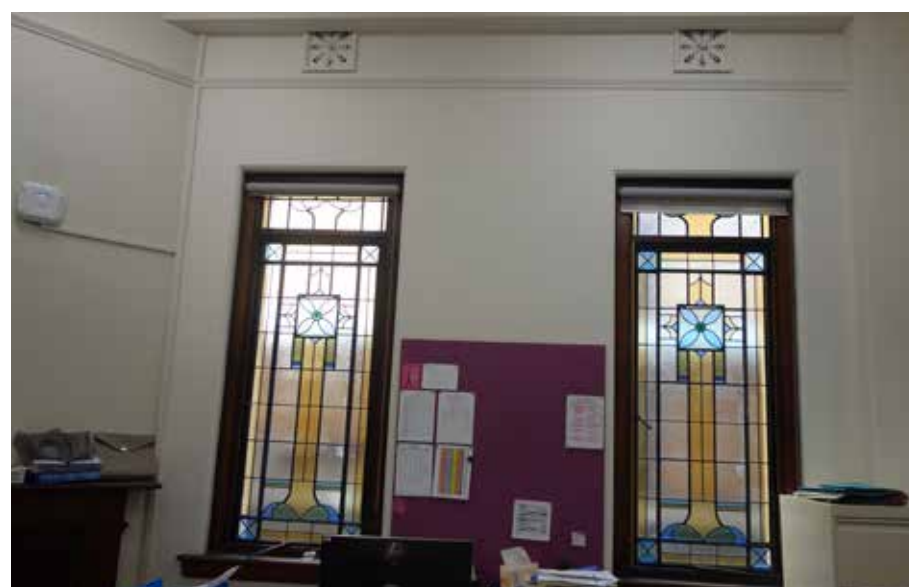
Figure 2.43: Original external wall vents of the Main School building are partially obstructed by the new false ceiling. Original stained glass windows on Level 2 face the courtyard between the Main Building and the Hughes Centre.
