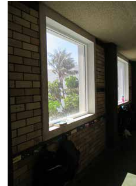
Figure 2.256: The former open balcony on the western side has been enclosed by a single pane of glass. Note the original exposed aggregate window surrounds.
