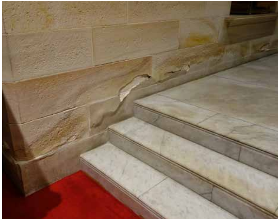
Figure 2.132: Image showing some of the blistering and erosion of the stonework from rising damp.
