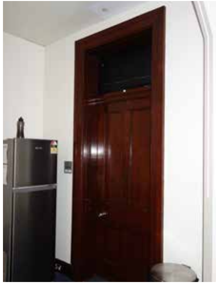
Figure 2.91: Original panelled door and architrave to the dorm accommodation on Level 4 of the South wing.
