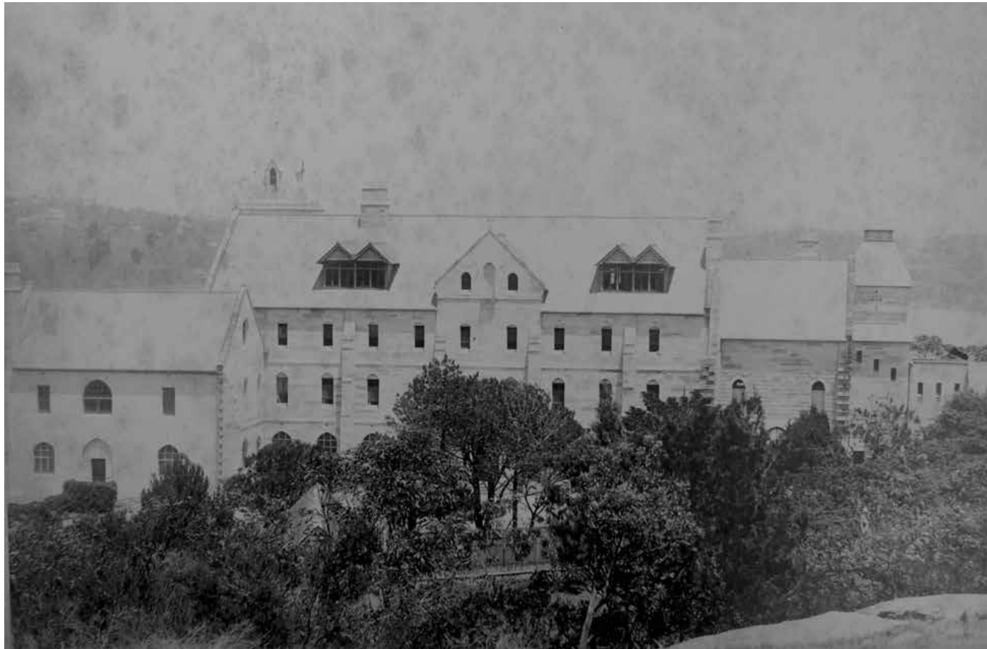
Figure A.46: The west and south wings on completion in 1888. This photograph recorded the east elevation. Provision was made in the uncompleted stone coursing for future additions for the chapel, and to the south wing. Source: Provincial Archives of the Society of the Sacred Heart (Album 11, Item 47)
