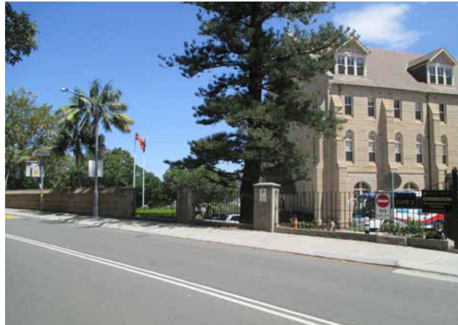
Figure 2.4: The sandstone boundary wall and modern aluminium fence panels on Vacluse Road just south of the Kincoppal exit gates.
