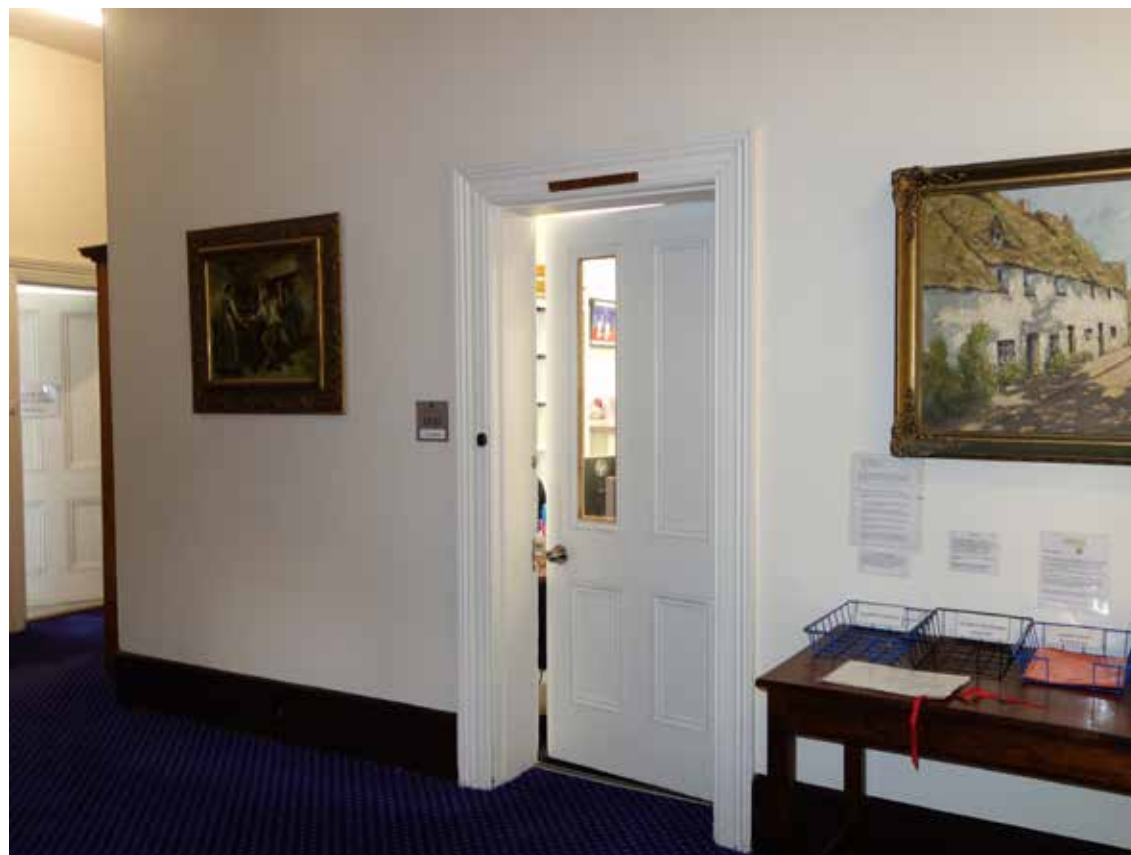
Figure 2.166: Typical timber panelled door and architrave at Level 3, dating from the 1882 reconstruction of Claremont by Hunt.
