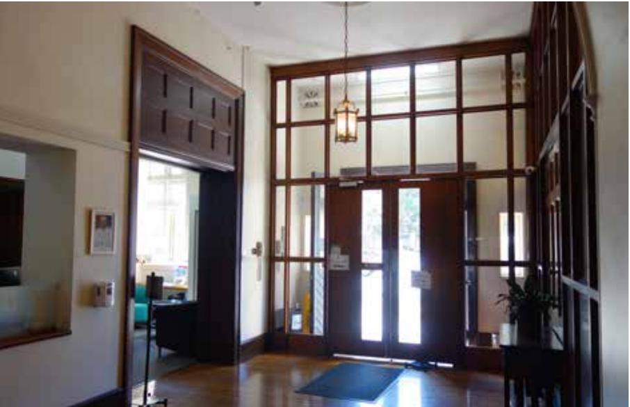
Figure 2.38: Main entrance foyer showing the modern timber partition (centre and right). The doorcase to the reception and waiting area on the left would appear to be original / early joinery.
