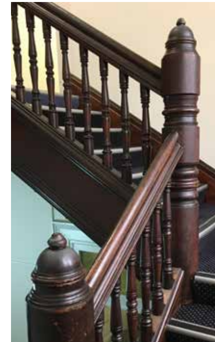
Figure 2.144: Detail of the turned balusters and newel posts of the staircase within Claremont.
