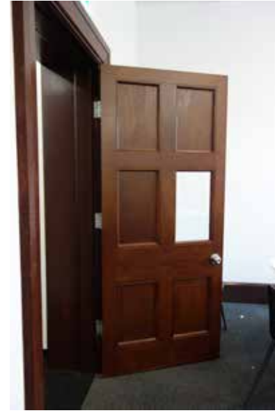
Figure 2.54: The original doors have been modified throughout to include a glass panel for security reasons.
