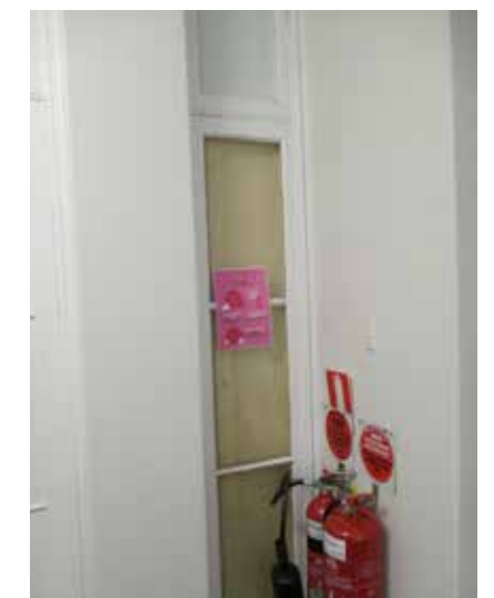
Figure 2.160: Detail of the fine glass French doors with side lights and timber panelled internal shutters from the corridor to the north.
