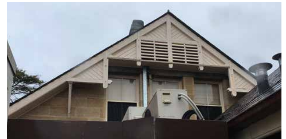
Figure 2.135: Timber gable bracket and screen on the northern elevation at Claremont.
