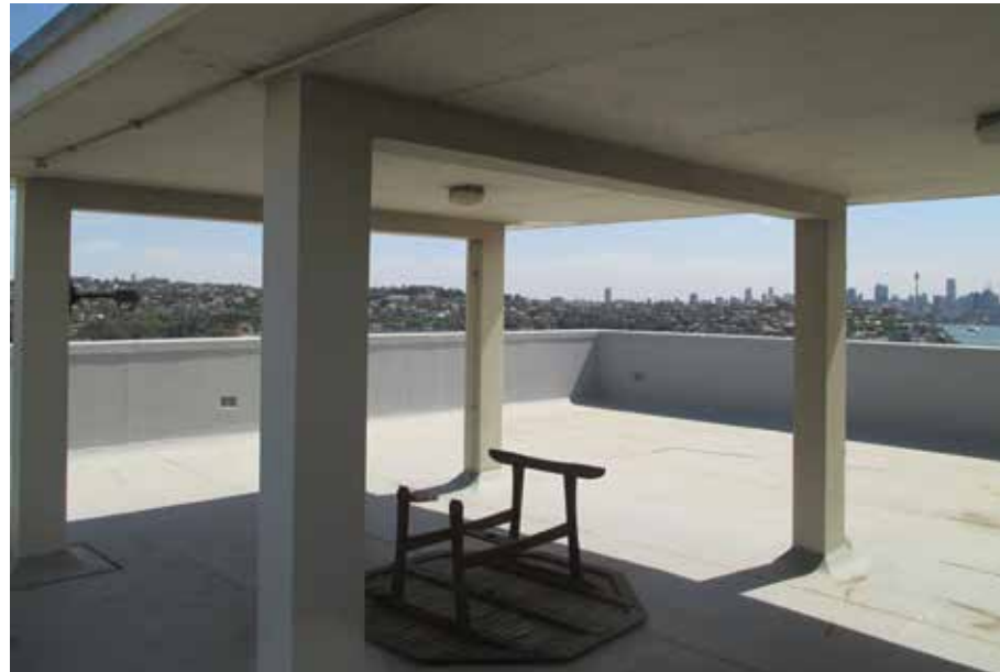
Figure 2.250: View south west over the harbour towards Rose Bay from the roof terrace at Barat Burn. Note the steel and concrete cantilevered flat roof.
