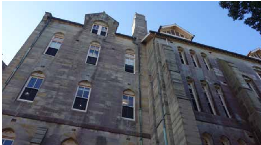
Figure 2.80: Junction between the 1888 wing and 1922 extension, marked by the setback and chimney. Note the different styles of dormer windows.
