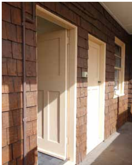
Figure 2.142: Timber shingled wall to the Level 3 verandah / balcony.
