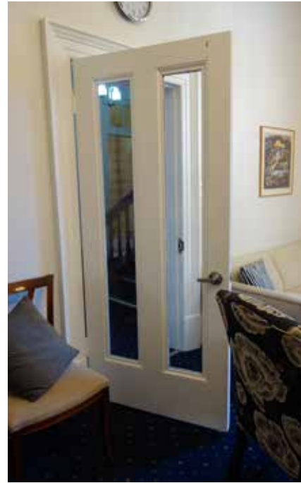
Figure 2.148: Typical door at Level 2 which has been modified with glass panels for security reasons.
