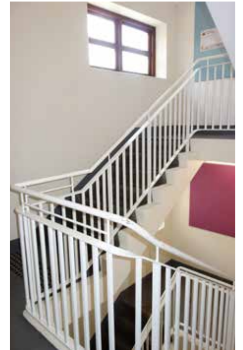
Figure 2.188: Concrete and steel fire stair at the southwestern corner of the building.
