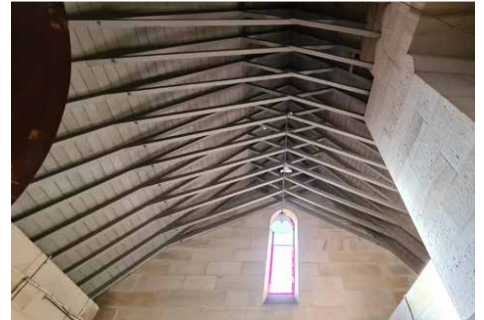
Figure 2.125: The exposed trusses in the Sacristan's Sacristy, similar to those in the Side / Stranger's Chapel.
