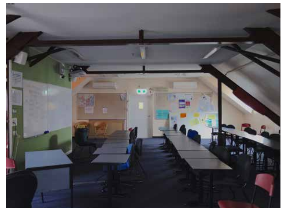
Figure 2.189: Level 4 / attic classroom with exposed steel ceiling trusses.
