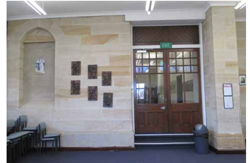
Figure 2.77: The interior of the 'verandah and balcony' on Level 2, looking towards the exposed sandstone wall of the main building and southern tower. The niche to the left in this image is one of the blind windows on the southern tower elevation. The exposed sandstone is evidence that this space was formerly an external space.
