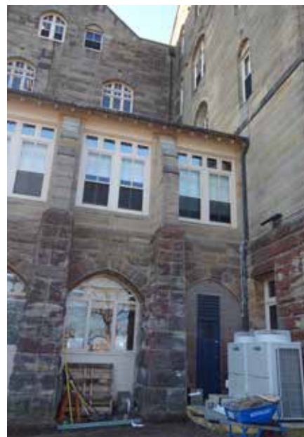
Figure 2.76: The eastern most bay of this elevation is infilled with masonry, rendered, lined and finished to resemble sandstone.
