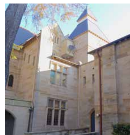
Figure 2.31: Northern tower of Main School Building and link to Claremont, seen from Chapel Square. The three stepped windows indicate a former stair.
