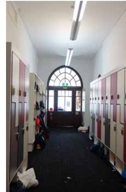
Figure 2.62: Many of the internal high level vents have been filled in on the corridor side, prohibiting natural cross ventilation. Image taken on Level 3 main corridor, looking north.
