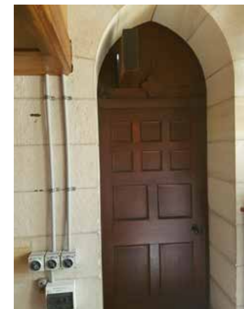
Figure 2.130: The panelled oak door as seen from the organ gallery and unsympathetic ductwork piercing through the panel above the door.
