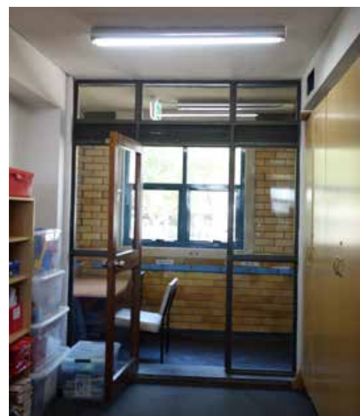
Figure 2.255: Steel framed door to balcony, showing the flooring finishes and terrazzo door threshold at Barat Burn.
