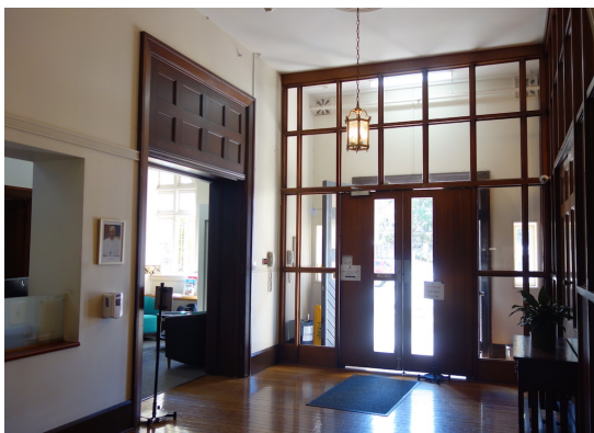
Figure 7.4.3: Main entrance foyer with modern glazed partition. The doorcase to the reception on the left appears to be original / early joinery.
