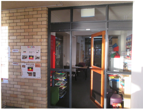
Figure 7.2.5: Original aluminium door and window set at Level 1, with modern timber glazed door.
