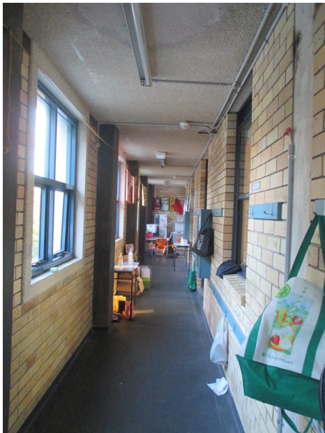
Figure 7.2.7: Former balcony at Level 1, showing modern aluminium window infill (LHS).
