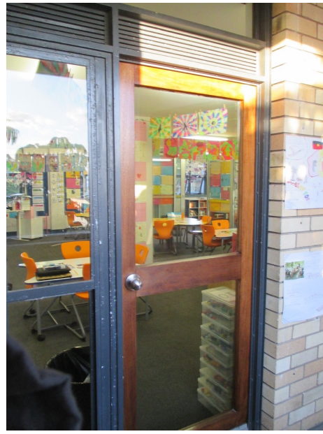
Figure 7.2.8: Original aluminium window and door set into former bedrooms off of the balcony on Level 1, with modern timber and glass door.
