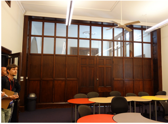
Figure 7.4.5: The classroom directly adjacent the main entry is separated by a 1990s timber partition, presented by the Year 12 students of that year. Surrounding this opening is original / early joinery, similar to the doorcase in the main reception area.
