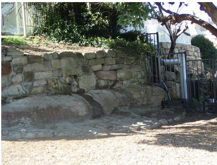
Figure 11. Precinct A: the retaining wall below the Early Learning Centre, sitting on sandstone bedrock
