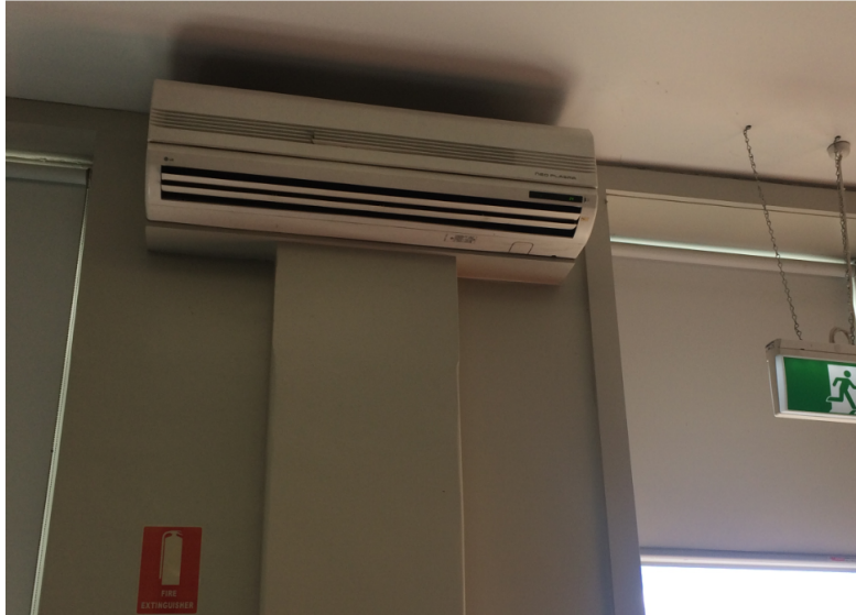
Photo 3.1.1 - Ground level wall mounted split
