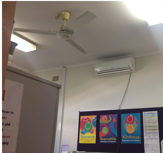
Photo 3.1.4 – Split A/C unit and sweep fan
