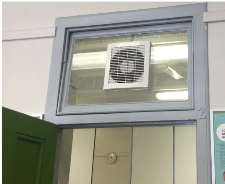
Photo 3.1.2 - Wall mounted fan to assist with “borrowed” ventilation
