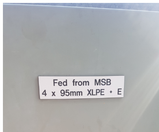
DB Located externally
