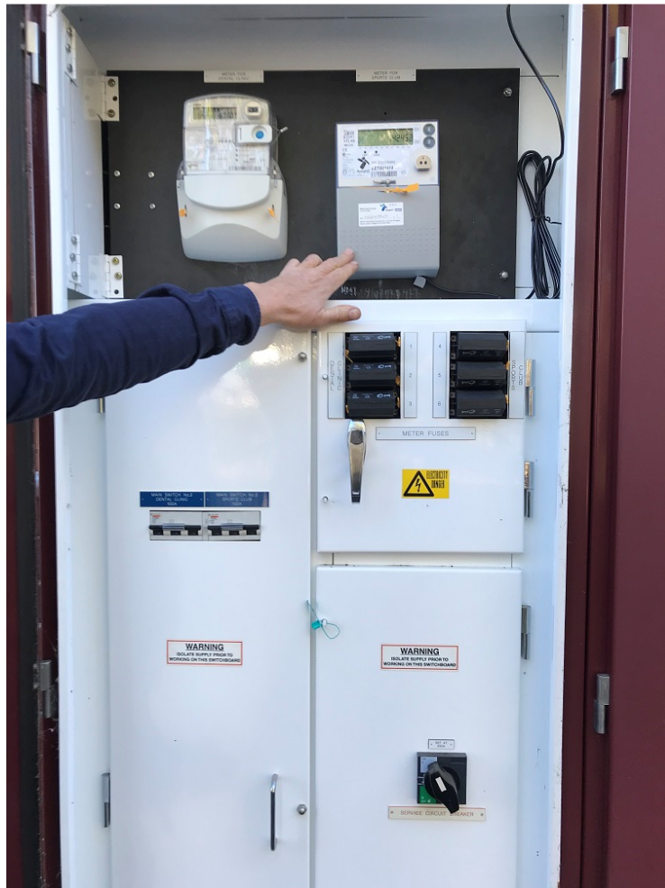
Main Switchboard Extension with 630A supply to school side configuration
