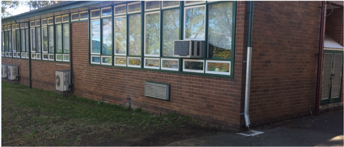
Photo 3.1.3 – Split and window mounted A/C units
