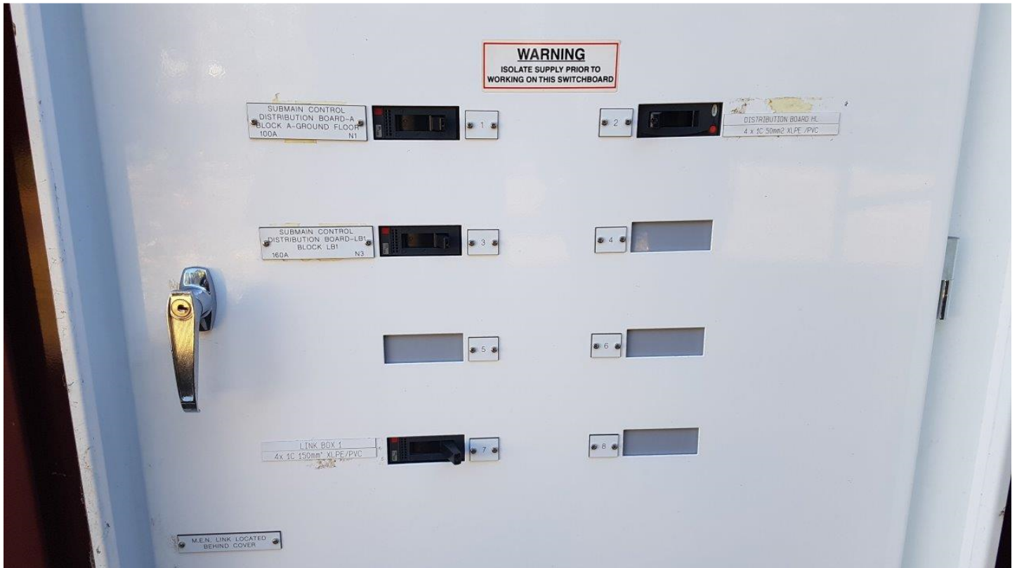
Main switchboard with 400A supply to school side configuration
