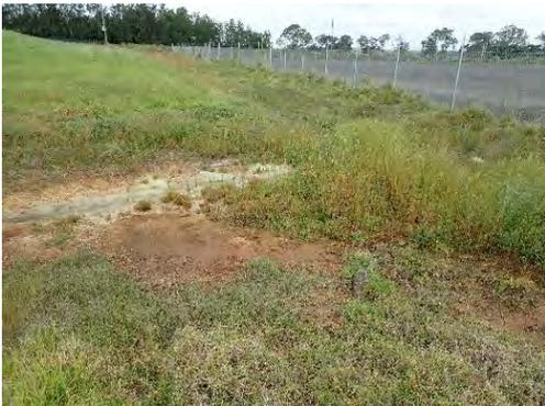
Figure 9 – Erosion exposure within embankment between hardstands. Aspect south
