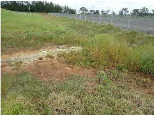
Figure 27 – Erosion exposure within embankment between hardstands. Aspect south
