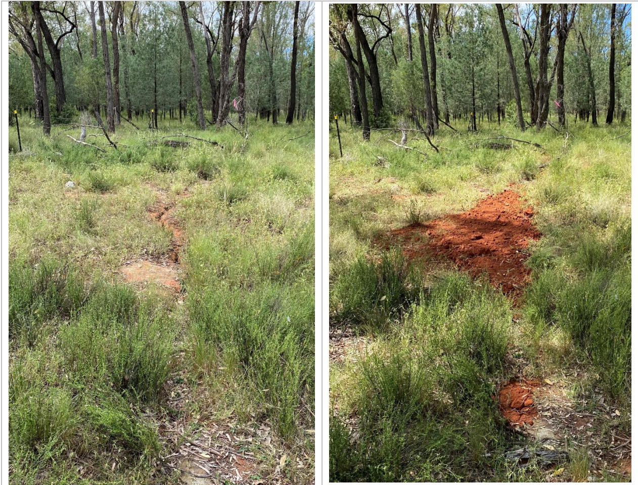
Figure A1-8 Photographs of Before and After Crack Remediation at the Narrabri Mine
