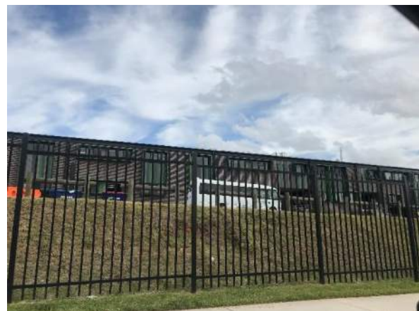
Figure 8: Completed building at St Francis Catholic College (Source: City Plan)
