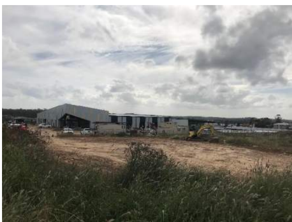
Figure 9: Buildings under construction at St Francis Catholic College (Source: City Plan)
