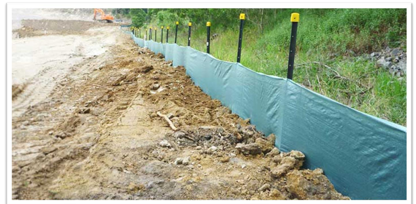
Figure 5 – Sediment Fence
