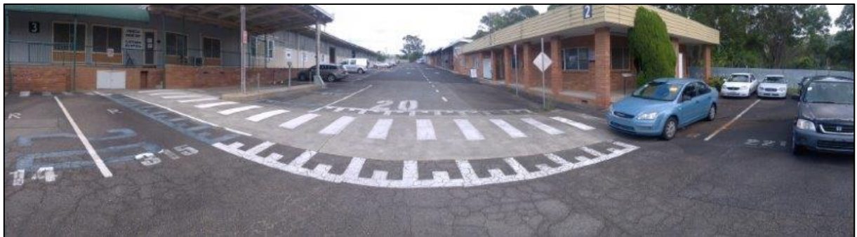
Figure 5 – Photograph from beyond the north-east corner of the site facing south-west, showing the former original UPSS area, with the former bowser island and awning visible. Some seepage discharging through the surface pavements at right side of photograph and down-slope of former UPSS. Some iron staining but no sheen visible on the seepage discharge.
