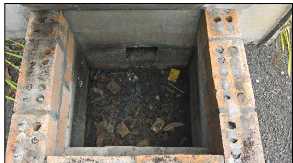
Figure 14 and Figure 15 – Photographs of the relatively small chemical store building, located adjacent to the southern site boundary. Inspection indicated some staining was visible on the concrete floor slab and that the store was designed to drain towards a small sump (pit – Figure 15) located externally on side of the building. The pit had fibre cement sheet (potential asbestos containing material) cover, that was observed to be in poor/average condition.
