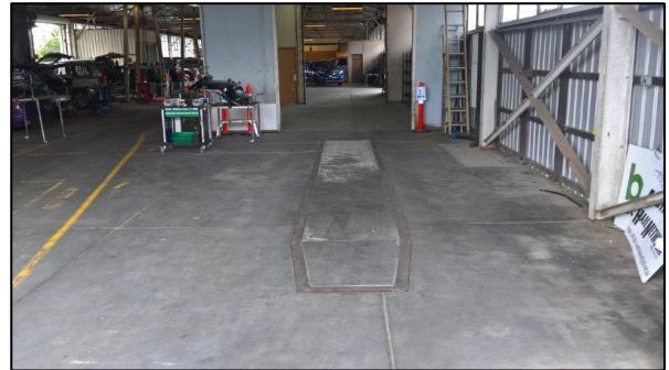
Figure 9 and Figure 10 – Photographs of the internal areas of the relatively large workshop, store and office building. Inspection identified signage that indicated past chemical storage, and oil filled equipment storage areas as well as an in-filled mechanics inspection pit. The building was being used as a hail-damage repair depot (paint-less dent removal) during the site walkover.
