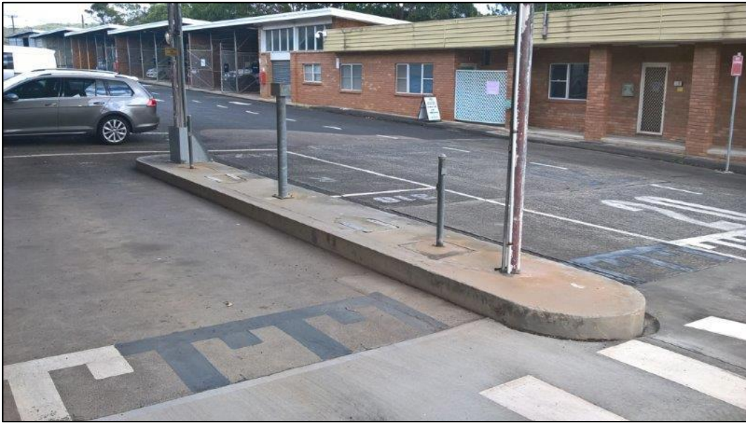
Figure 6 – Photograph of the original UPSS bowser island. The site boundary appears to bisect the former UPSS area. Inspection identified the former bowser plinth and two possible vent lines. No former dip or fill points were identified in the mapped location of the former UPSS. Hazardous chemical records search results indicated that this area historically comprised a single bowser island, with two bowzers and four USTs (north-west (right side) of bowser island).
