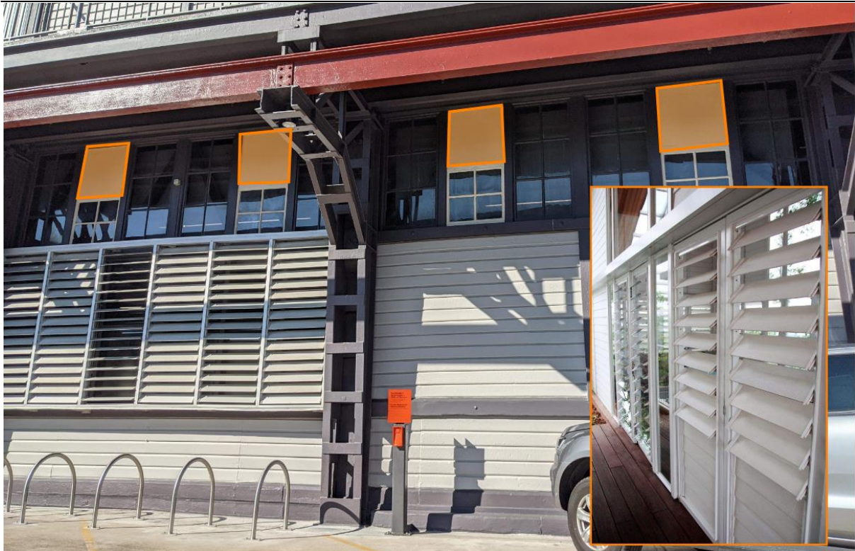
Figure 11: Ground floor high level FC panels to western façade. Right: Example of proposed operable louvres to be painted to match colour of existing FC panels. Extracted from ARUP report Wharf 4&5 – Dance Studio Ventilation dated 28 May 2021.
