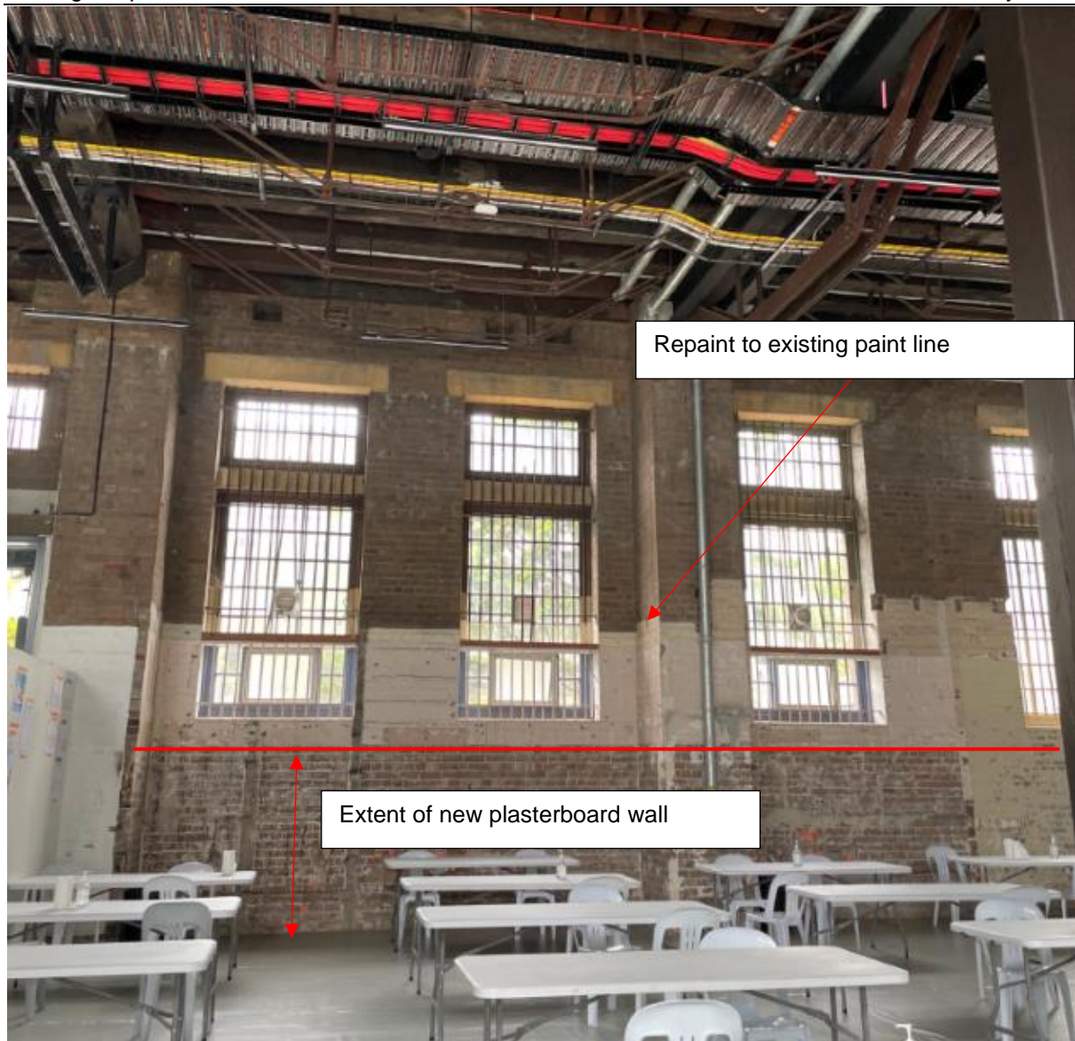
Figure 22: Southern brickwall to Commercial 3. Note lower section previously chased for services and damaged brick face where previous tiles removed
