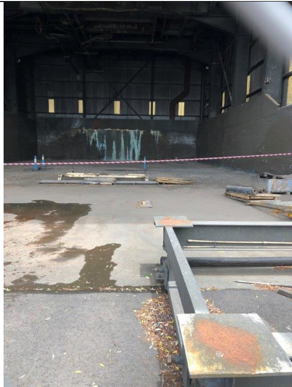
Photograph 3 Copper staining visible on internal surfaces of site buildings
