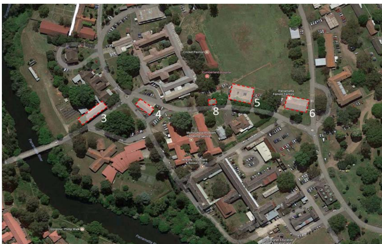
Figure 2-5 Five buildings in Cumberland East to be demolished (basemap: Google)
