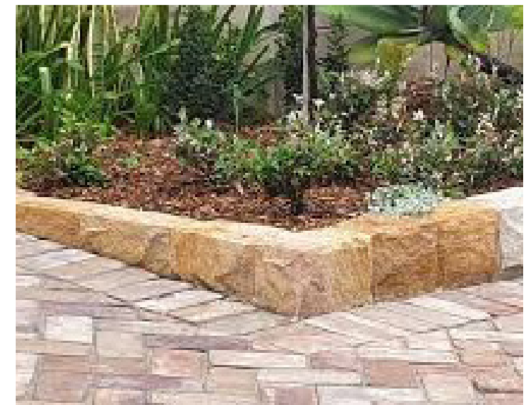
Brick Paving and Sandstone Edging
