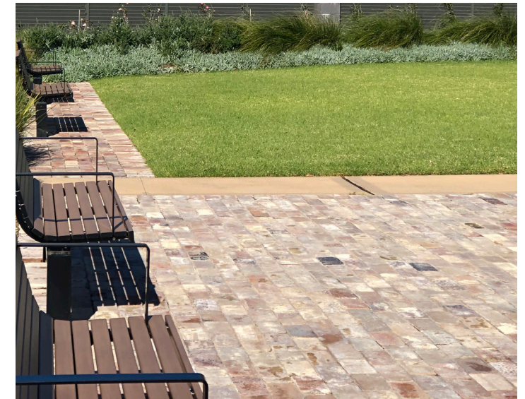
Recycled Brick Paving
