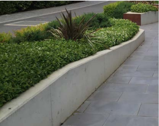
Off-form Concrete Retaining walls (up to 900mm)
