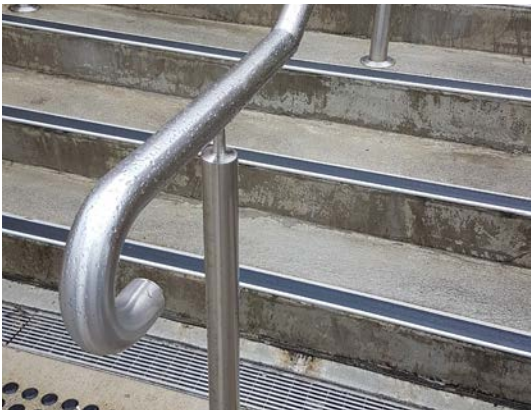
Stainless Steel Handrails to AS1428
