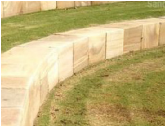
Curved Sandstone block seating wall
