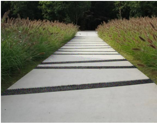
Large Angular Poured Concrete Paving
