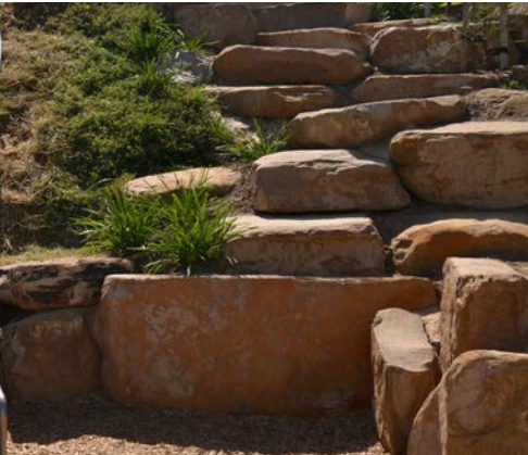
Sandstone Log Embankment with Gravel infill and Planting
