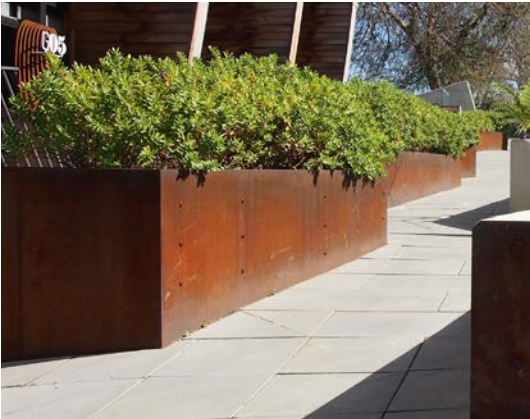
Corten Steel Retaining walls (up to 600mm)
