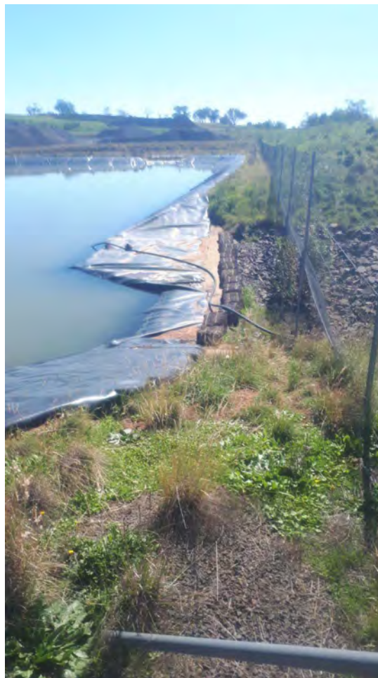
Figure 2: Picture of water storage dam taken 14 April 2020
