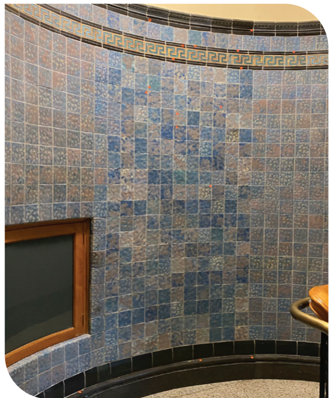
Infilled wall with salvaged and new.
