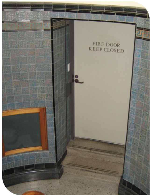
Stairwell with 1960s openings.
