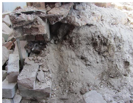
Figure 6.2: View of building foundation with sandy loam fill (Photograph by J. Norfolk, 18 January 2019)
