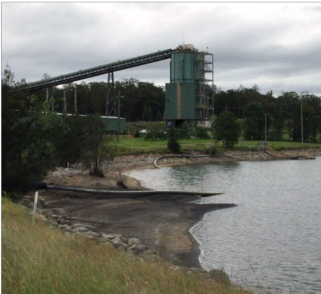
b) Looking northeast - Train Shed, Conveyor, Coal Bin and Rail Loop Dam.
