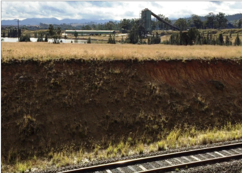
a) Distant view of Rail Loop Dam, Train Shed, Coal Bin and Conveyor - looking northwest.
