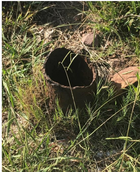
Plate 3 Condition of Groundwater Monitoring Bore GW078135 (Photo dated 14 March 2019)
