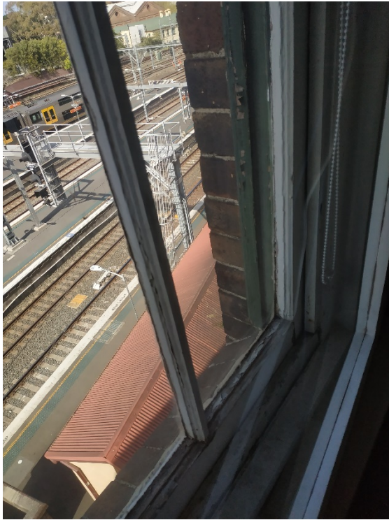
Figure 14 Window framing on southern side of second floor of 125-127 Little Eveleigh Street showing consistent sill and frame without cracks or crevices
