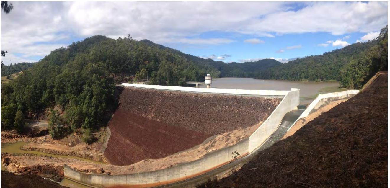
Figure 5: Panoramic view of spillway (foreground), dam wall, and intake tower (background)
