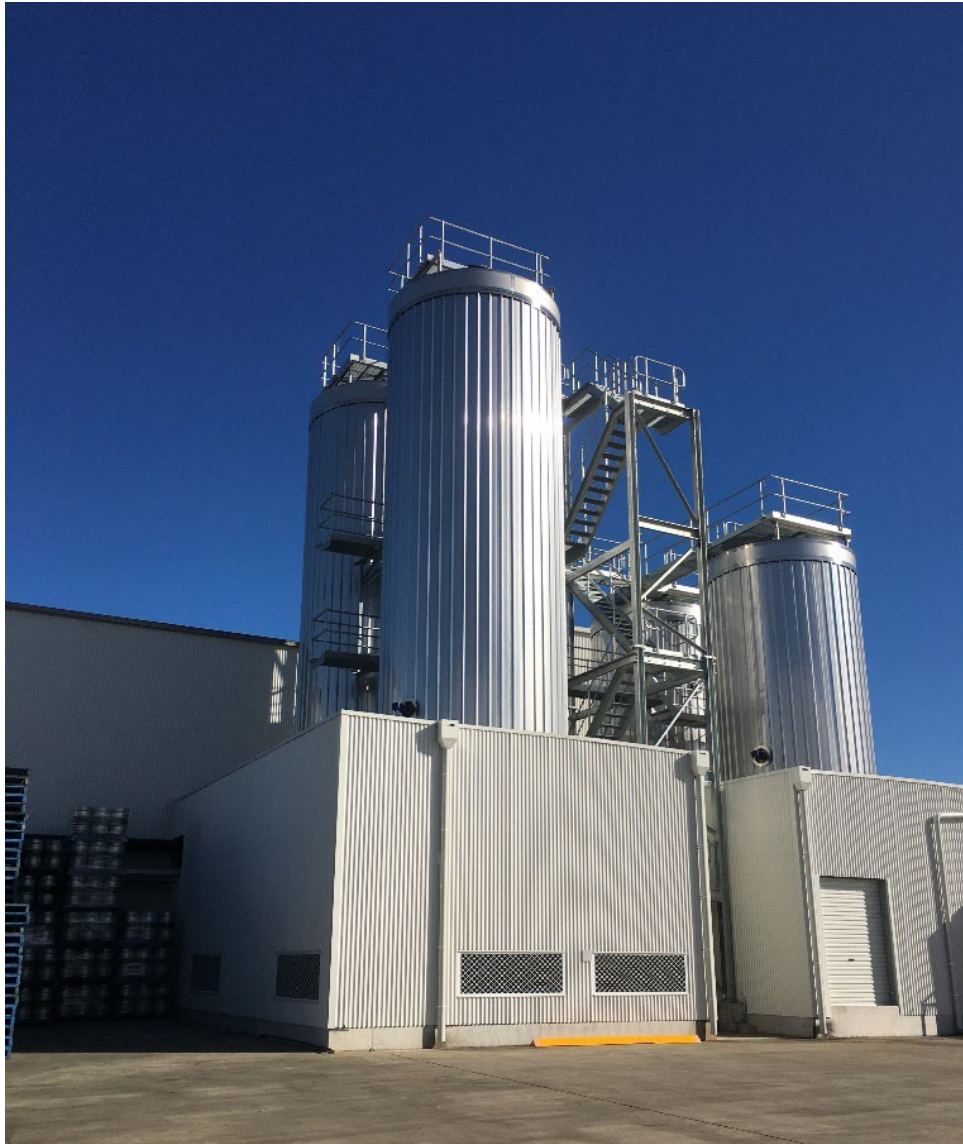
Photo 1 Existing 400HL Bright Beer and 800HL Fermenter tanks (16m height) at Kite Crescent brewery
