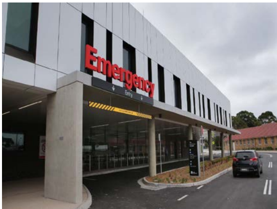
The entrance to the Emergency Department, part of the completed Sutherland Hospital redevelopment
