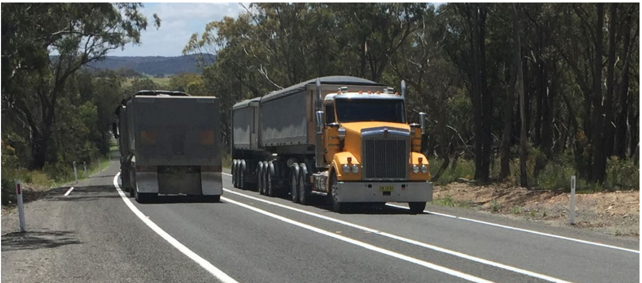
Photograph 2.4 Trucks passing on Brayton Road – wide centreline treatment increasing the separation distance (November 2020)
