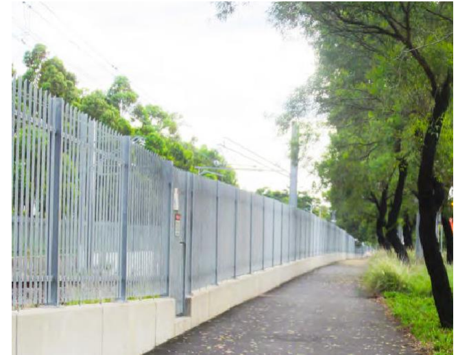
Homebush, Sydney. Rail corridor security fences should be robust, easily maintained, modular systems that are readily integrated with other urban design elements such as retaining walls. (Source: AECOM)
