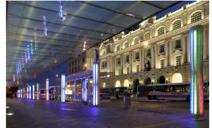
Britomart Transport Centre, Auckland. Lighting is designed to provide a safe, legible and comfortable environment for customers and users. (Architects: Mario Madayag & Jasmax. Source: Opus)
